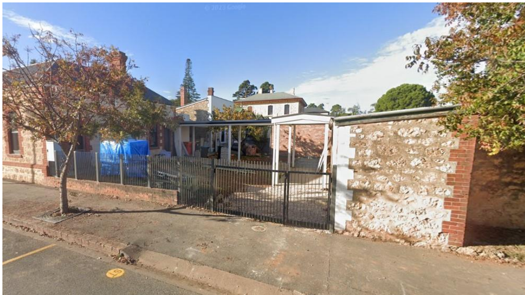
Shops and stables during conservation works in 2023.
