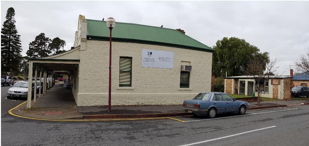
Shops with converted rear stables prior to conservation works in 2019.
