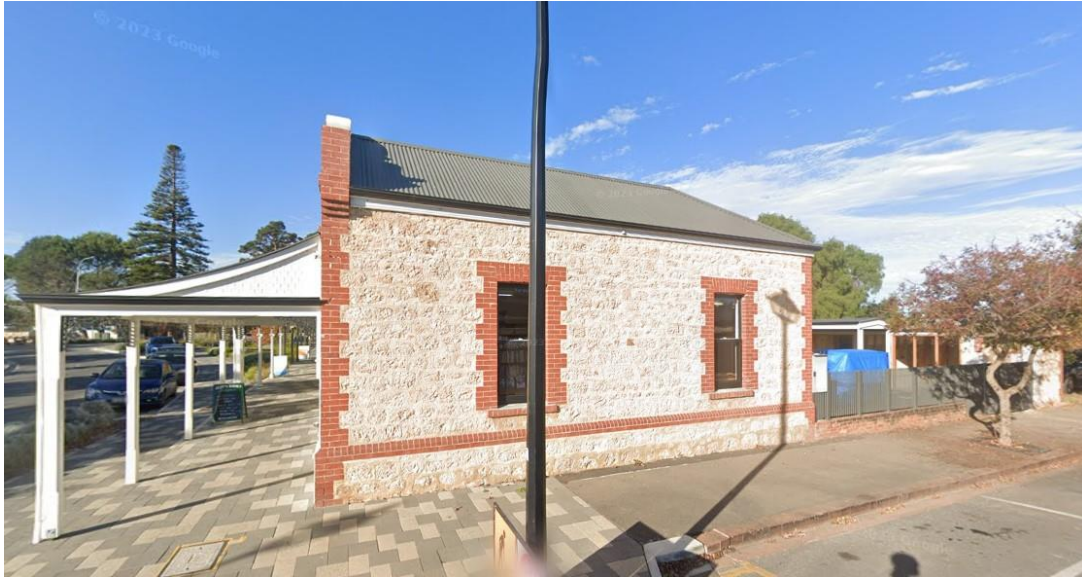
Shops from the corner of Catherine Street and Albyn Terrace during conservation works in 2023.
