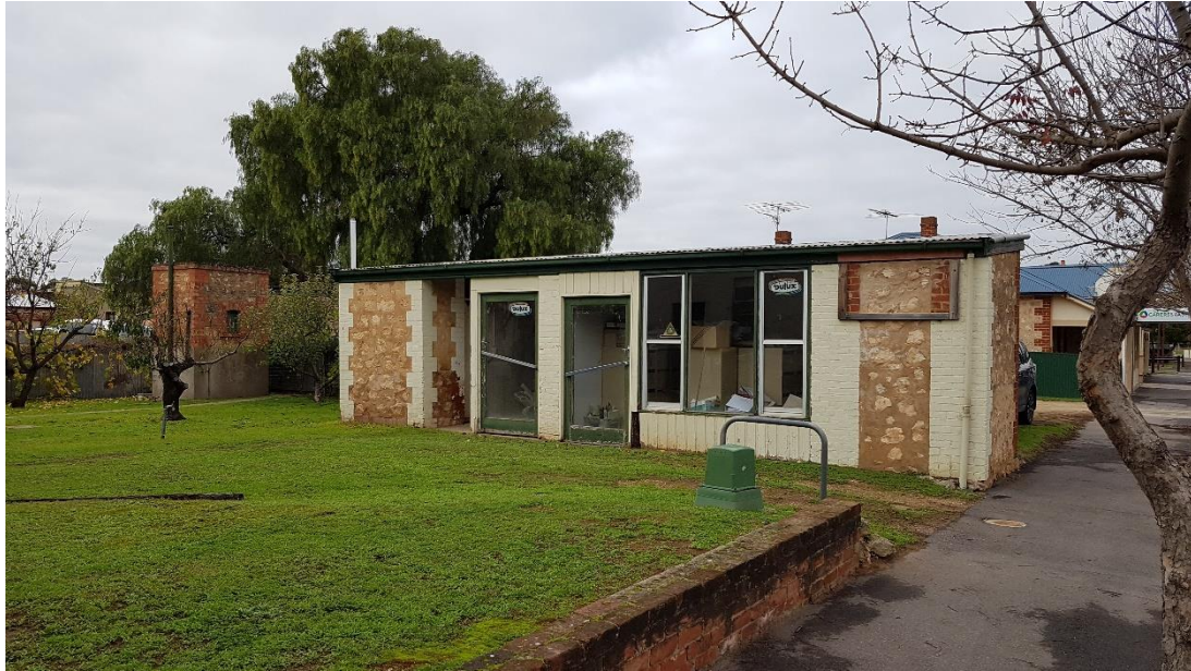
Stables at the rear of the site prior to conservation works in 2019.
