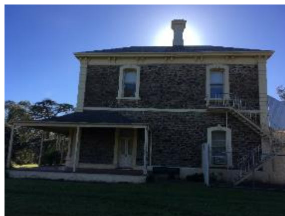
Lochiel Park House, south-western elevation
