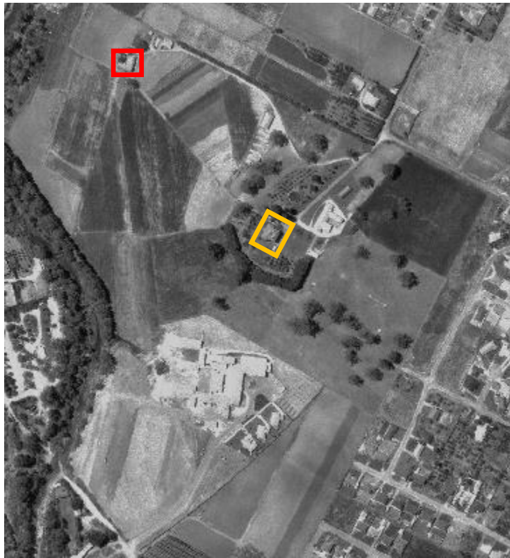
Aerial Lochiel Park Training Centre 1969, note construction of Brookway Park (junior boys reformatory) lower centre of image
