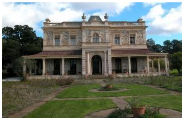
'Para Para' House, Gawler (SHP 10057)
