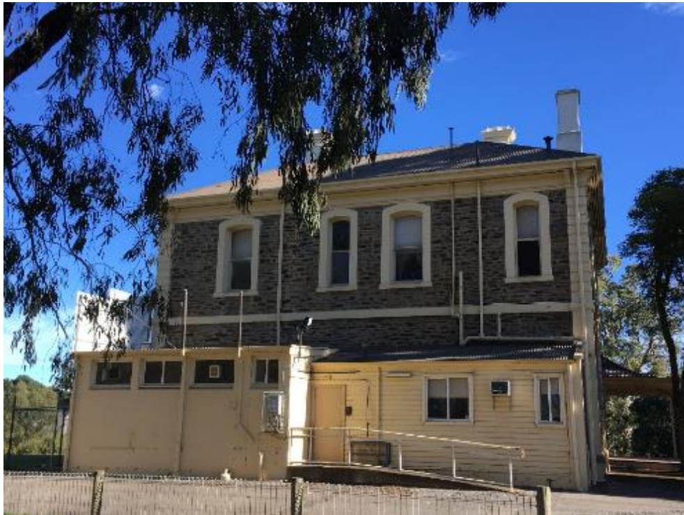
Lochiel Park House, rear elevation
