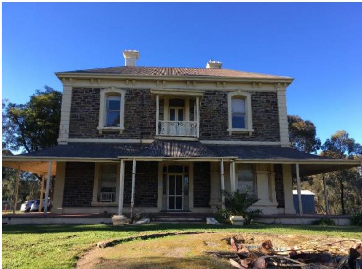
Lochiel Park House, front elevation
