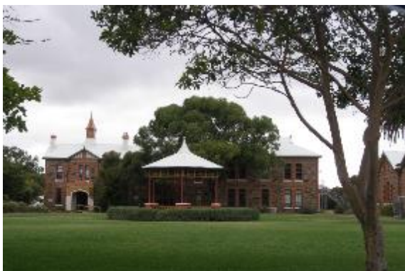
Minda Rogerson Building (SHP 14474)
