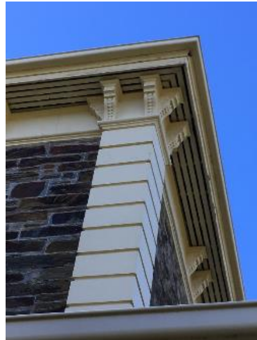
Detail of eave, quoins and dentils
