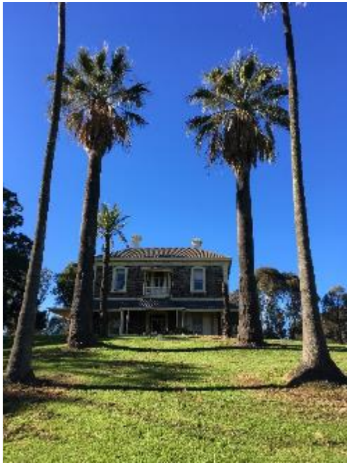
View to front of house from Palm Avenue, note the broken palm mid-right
