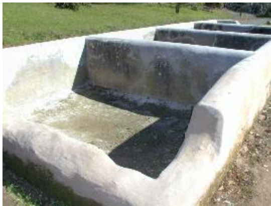
Manure Pits, Brownhill Creek Recreation Park (SHP 14782)
