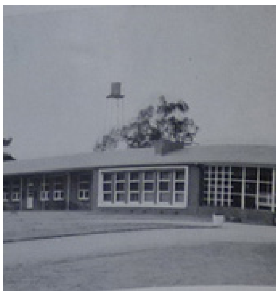
Lochiel Park dormitory and kitchen – built 1958 and demolished mid-1990s
