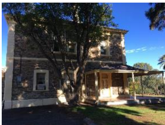
Lochiel Park House, north-eastern elevation
