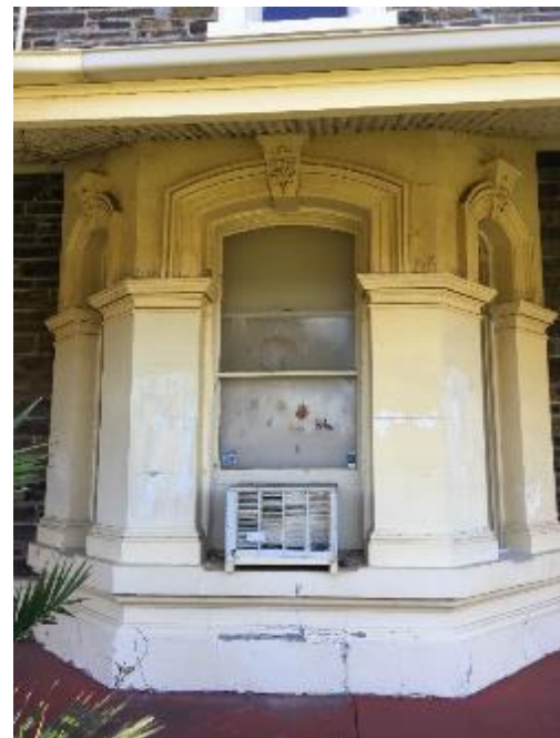
Detail of Bay window, note window-mounted air conditioning unit
