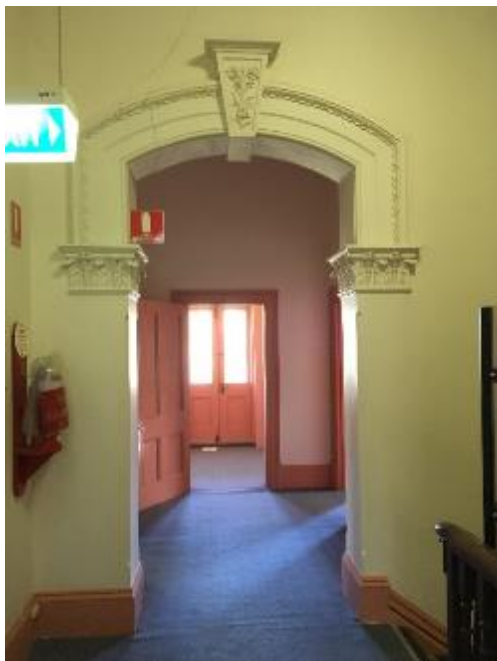
Detail of larger arch, first floor
