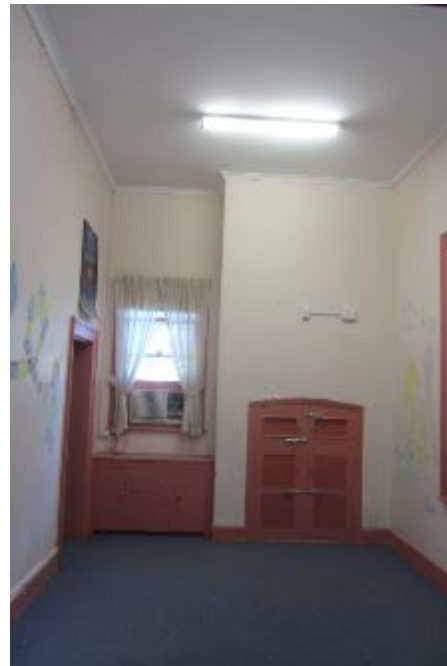
Kitchen (refitted), note fireplace has been enclosed
