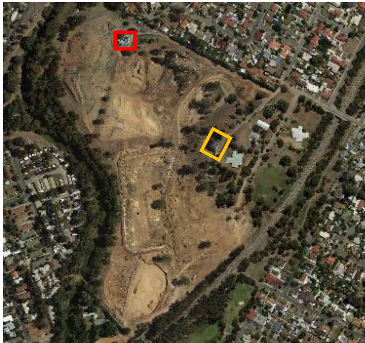
Aerial Lochiel Park 2007, showing extensive land clearing and excavation in preparation for new sustainable housing development, note demolition of 1958 accommodation/kitchen block
