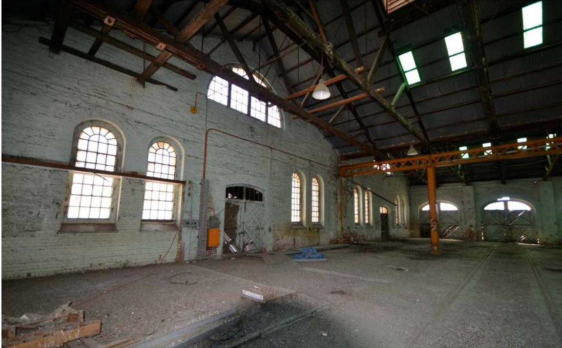
Old Bulk Store – Interior – note original central metal web truss and support columns
