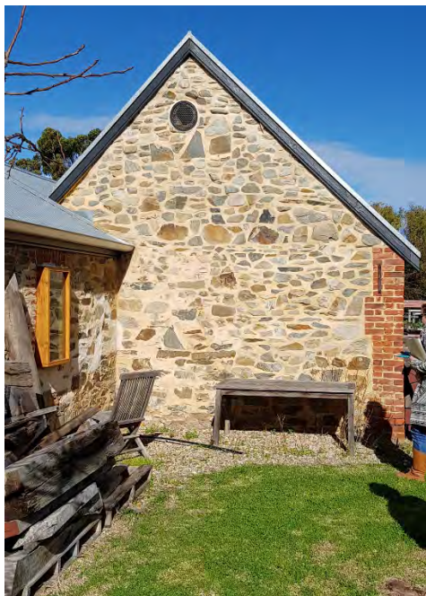
North elevation. Note gable end with random bluestone stonework with redbrick quoin. July 2017 Source: DEW
