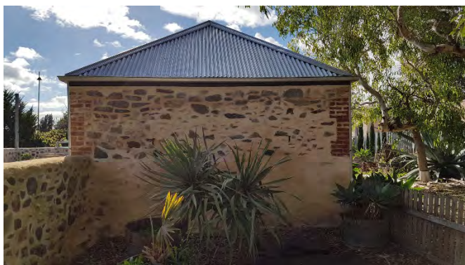
South elevation. Note bluestone and redbrick construction at the top of the wall with render below. July 2017. Source: DEW
