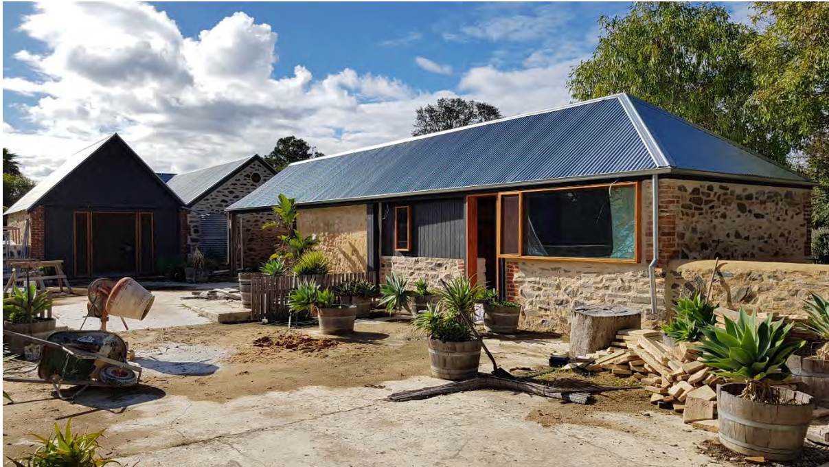
Middleton Mill outbuildings. July 2017
