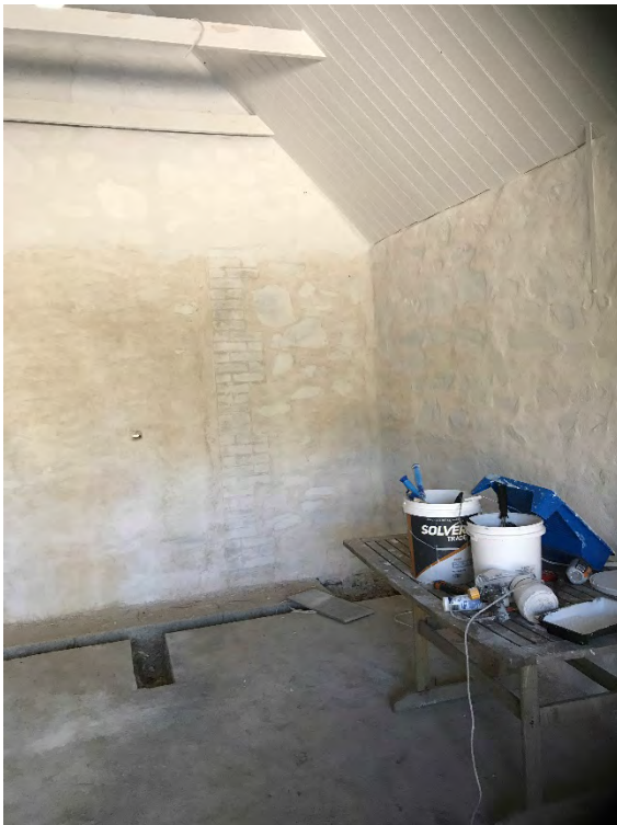
Interior of mill outbuildings showing lime wash walls. (2017) Source: DEW
