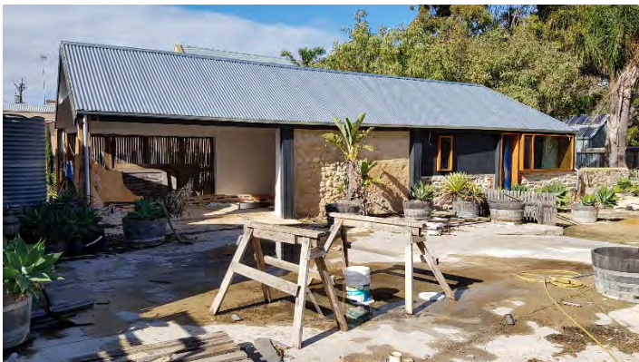
West elevation of Building 2 (stable). Note limestone panel with open end kitchen area and half-height bluestone walls. July 2017. Source: DEW
