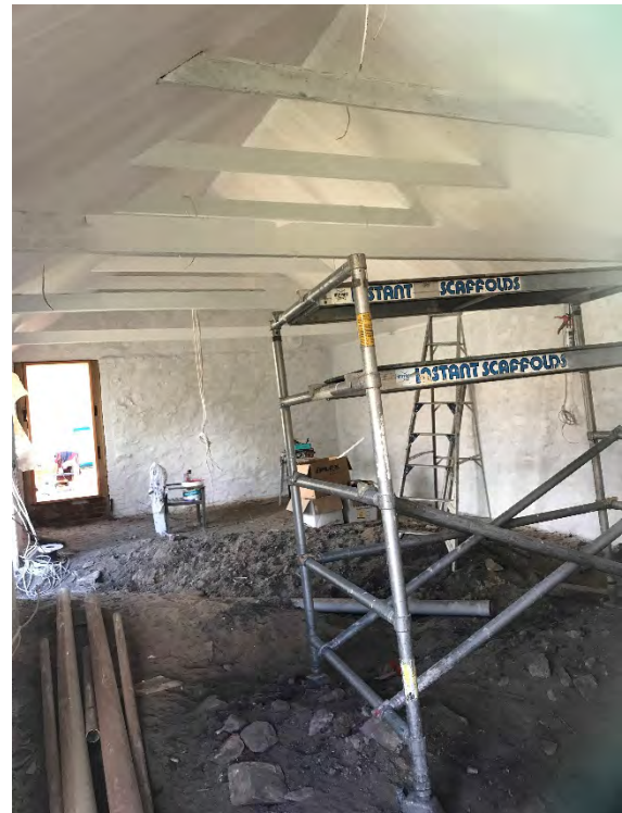
Interior of mill outbuildings showing lime wash walls, exposed trusses and ceiling panelling. (2017) Source: DEW
