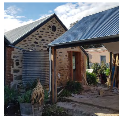
Open-ended kitchen area. July 2017. Source: DEW
