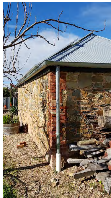
North elevation. Note hipped roof. July 2017 Source: DEW
