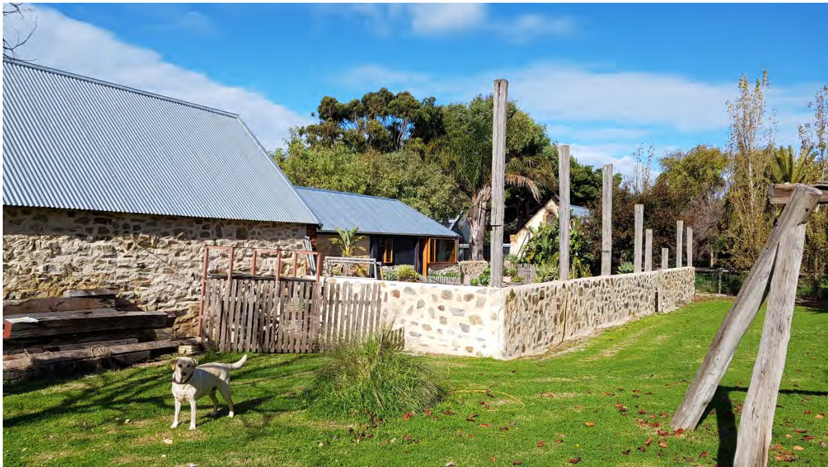
West elevation. Note low stone wall built c2017 by the current owner. July 2017
