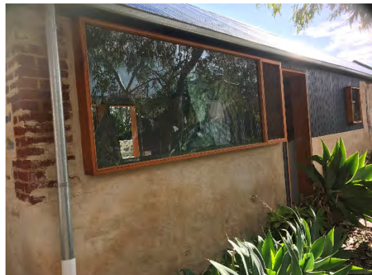
East elevation of Building 2. Note half-height walls with windows and timber panelling above. July 2017. Source: DEW
