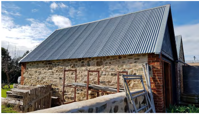
West elevation. Note double gable ends of the south side of the building with timber infill and bluestone cladding. July 2017 Source:DEW
