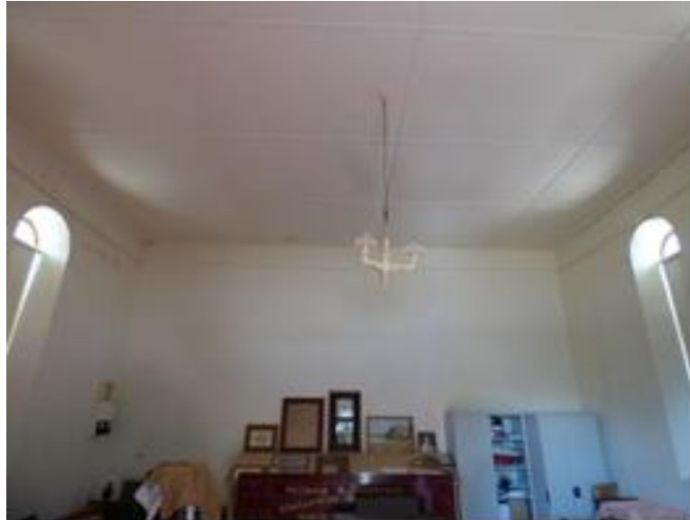
Internal view Former Milang Primitive Methodist Chapel Note ceiling and arched windows.
