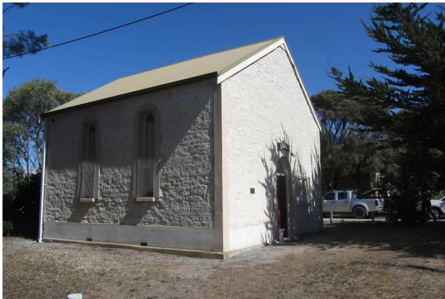
Former Milang Primitive Methodist Chapel external view. Note rendered base of walls and rendered corners.
