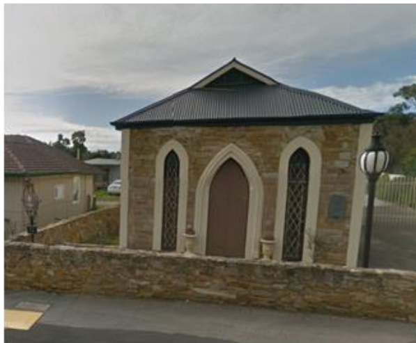
27 High Street, Willunga, 1867, LHP Note the non-original front windows and doors. Photo Source: https://www.instantstreetview.com/
