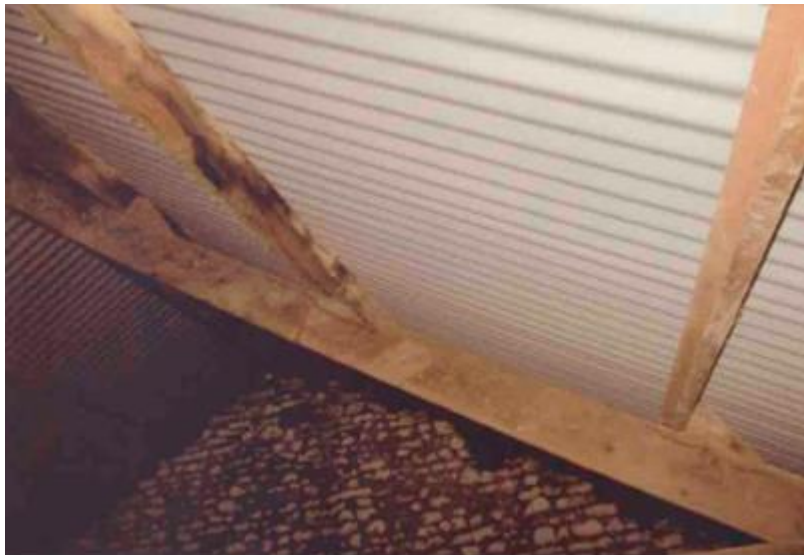
Former Milang Primitive Methodist Chapel Internal view illustrating roof framing.
