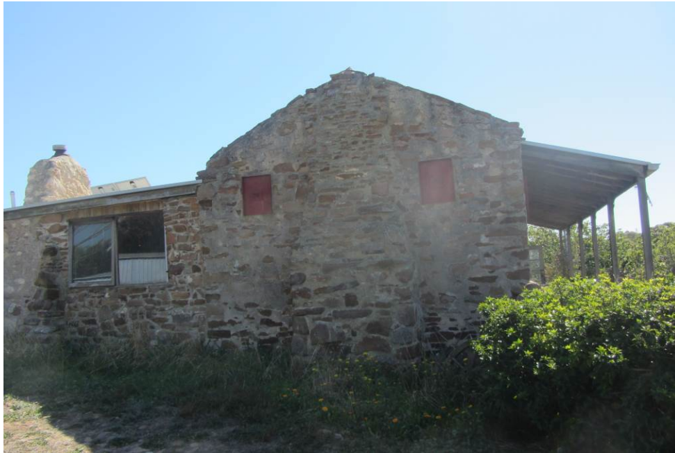
Whittle Farmhouse southern façade. Note the partially-constructed chimney, the restored lean-to kitchen, extensive use of concrete to repoint the stonework and the bracing plates.
