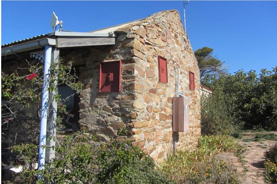
Whittle Farmhouse, north-east corner of the building where the most substantial cracking had occurred. Note the extensive use of concrete to repoint the stonework and the metal plates.
