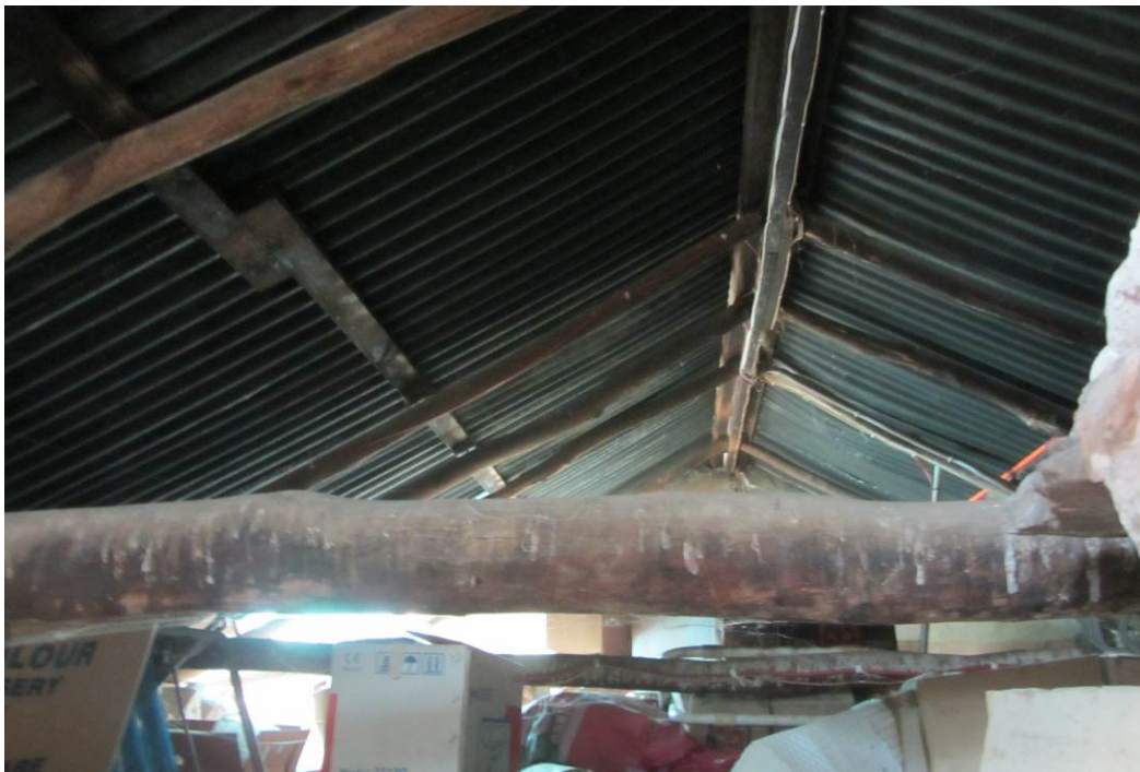
Whittle Farmhouse, roof frame. Note the use of bush and sawn timbers.
