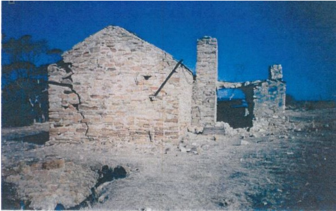
Whittle Farmhouse view from the north, 1994, prior to restoration. Note the substantial cracking, chimney, addition and well in the foreground.
