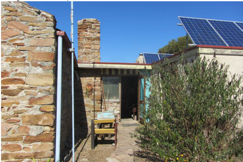
Whittle Farmhouse view to the south. Note the chimney and the restored lean-to kitchen and new addition.
