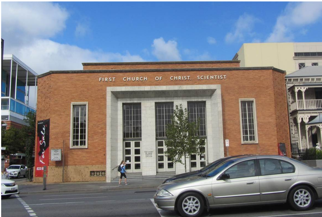
First Church of Christ. Scientist church- North Elevation- April 2017. Note the chamfered corners, marble portico, vertical windows, cornice, Roman lattice and set back plant room.
