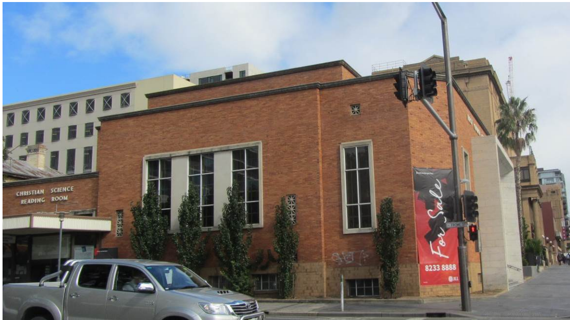
First Church of Christ. Scientist church- East Elevation- April 2017. Note the vertical windows with concrete window surrounds, basement windows and reading room.
