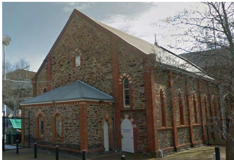
The Hindmarsh Historical Society Museum (former Hindmarsh Fire Station & Christian Chapel SHP13693, (1846)
