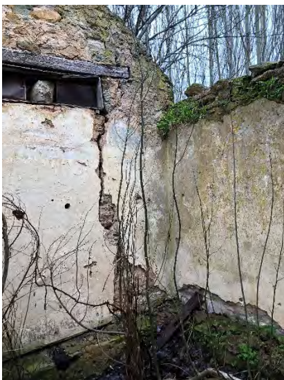
Inside the gabled porch, showing blocked in door and missing roof. August 2018 Source: DEW
