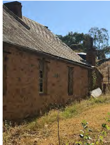
South-west elevation note the stone and brick chimney at the rear. (March 2018) Source DEW
