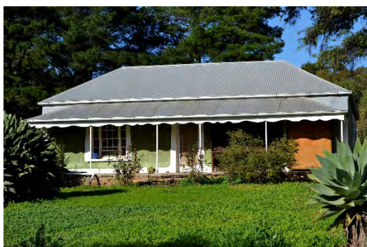
Dwelling Buckland House Sometimes School, 21 St Lukes Street, Willunga, 1840, SHP14165 (2016) Source: DEW
