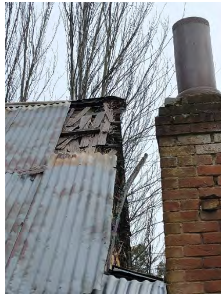
Roof of the chapel showing missing sheet of iron and original timber shingles underneath. August 2018 Source: DEW
