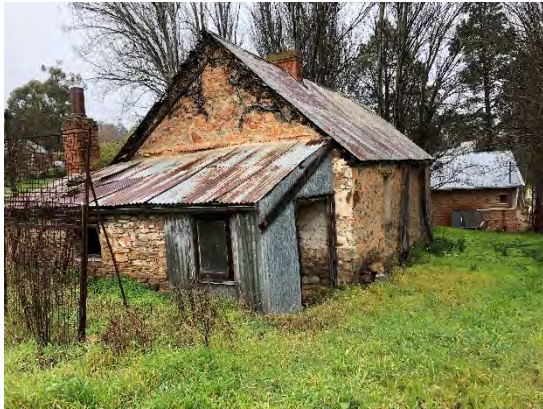
Rear of the chapel showing the cgi-clad section with side door and window. August 2018 Source: DEW
