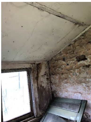
Interior of the cgi clad section of the lean-to. Note lime-washed stone and timber particle board cladding. (August 2018) Source: DEW
