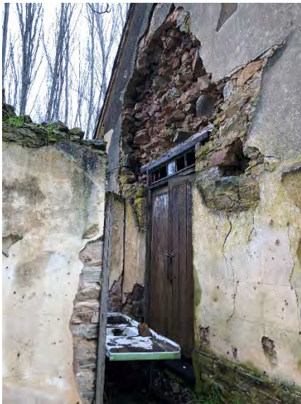
South-west end of the chapel showing missing render and stone work underneath. August 2018 Source: DEW
