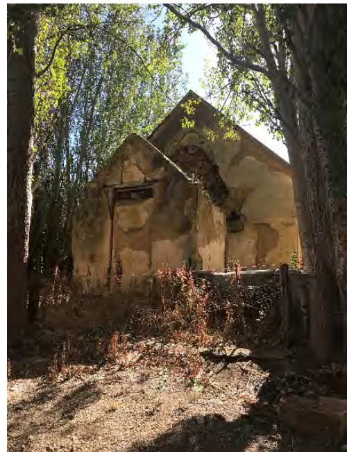
Front wall of the chapel. Note the rendered stone work and bricked up front door. (March 2018) Source DEW
