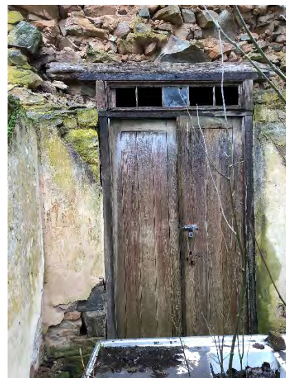
Front door, showing original lintel and transom. August 2018 Source: DEW
