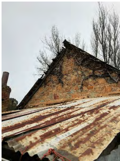
Rear gable. Note missing bargeboard and remnant ivy. (August 2018) Source: DEW
