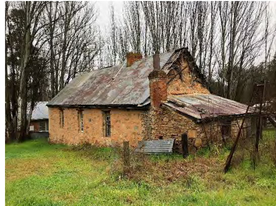
Rear of the chapel showing the stone section with red-brick chimney and window. August 2018 Source: DEW
