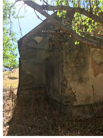
Front corner of the chapel. Note the crumbling render and stone work underneath. (March 2018) Source DEW
