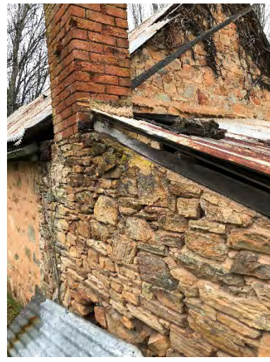
Stone lean-to at rear of the church. Note missing pointing, red brick chimney. (August 2018) Source: DEW
