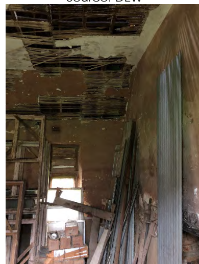
Interior of the main body of the chapel showing the internal dividing wall and top of the fire place to the right. Note lath and plaster ceiling. (August 2018) Source: DEW
