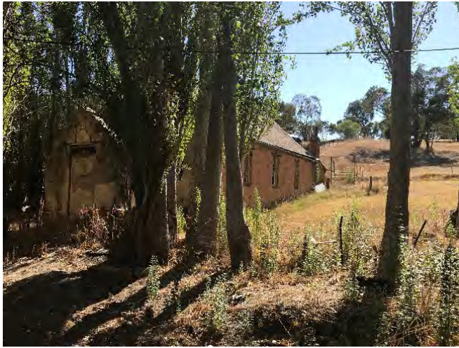
South-west elevation of the Houghton Union Chapel. Note the three-bays of windows and siting into the hill. (March 2018) Source DEW
