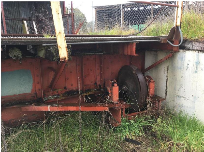
**Wheel and outer rail that enabled operation without balancing the locomotives**
