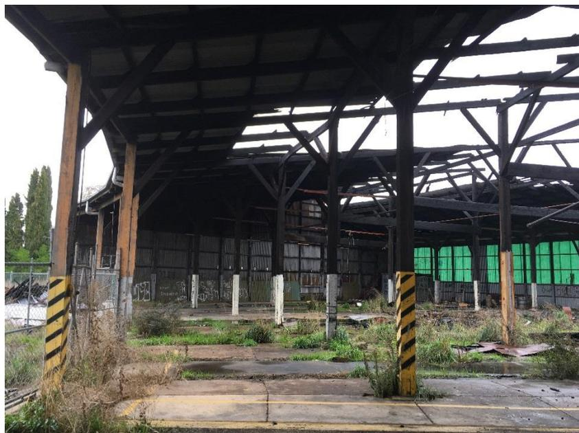
**Roundhouse view to south showing intact and undamaged posts at front of structure**
