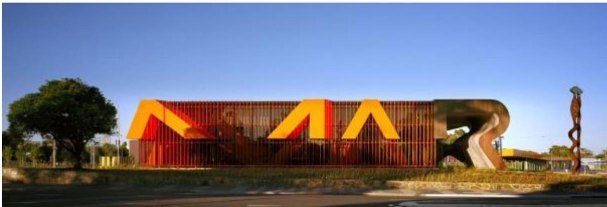
**Marion Cultural Centre, north-eastern elevation facing Diagonal Road. MAR are created from a steel framework clad in steel plate, copper plate and timber batons. Note the grille and sculpture I in the adjoining landscape.**
