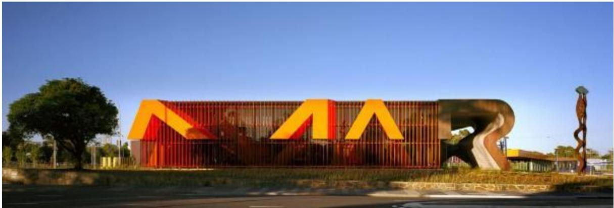
**Marion Cultural Centre, north-eastern elevation facing Diagonal Road. MAR are created from a steel framework clad in steel plate, copper plate and timber batons. Note the grille and sculpture I in the adjoining landscape.**
