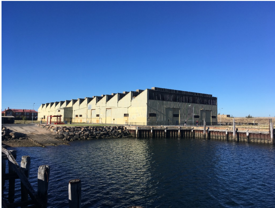
Shed 26 showing southern and western elevations
