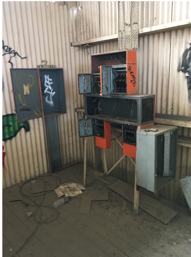
Shed 26 example of remnant machinery
