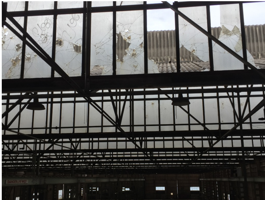
Shed 26 note the broken glass in the northern lights and hood on the ridgeline.
