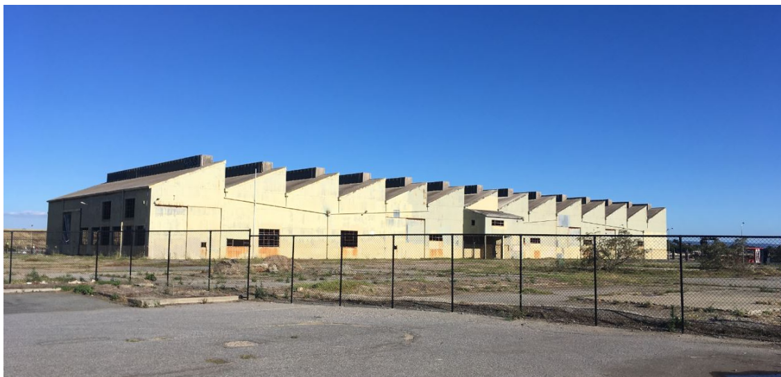
Shed 26, view of western and northern elevations
