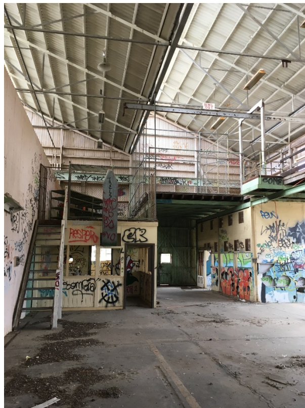
Shed 26 showing the mezzanine level and spaces below.
