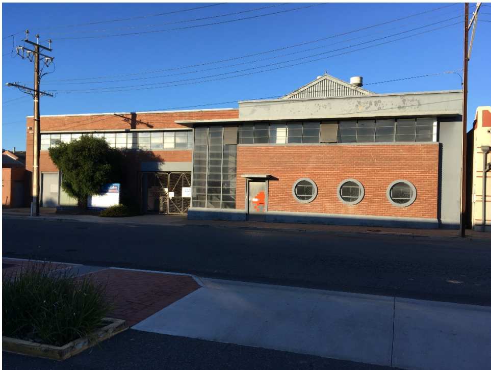
Former BALM Paints Duco Plant, 75 Lipson Street
