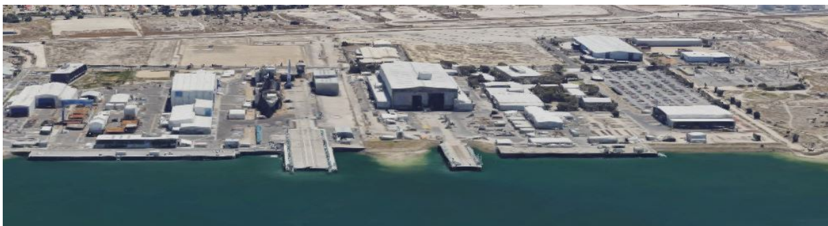
Australian Submarine Corporation facility at Osborne
