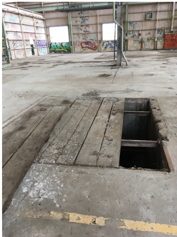
Shed 26 showing an inspection pit.
