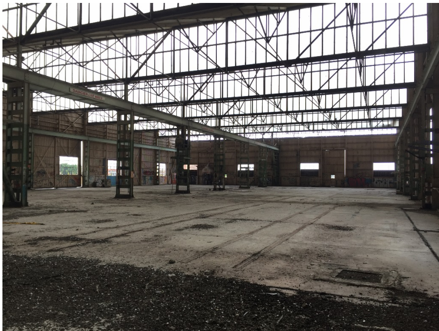
Interior of Shed 26 note the crane gantry, rail lines and infilled sumps.
