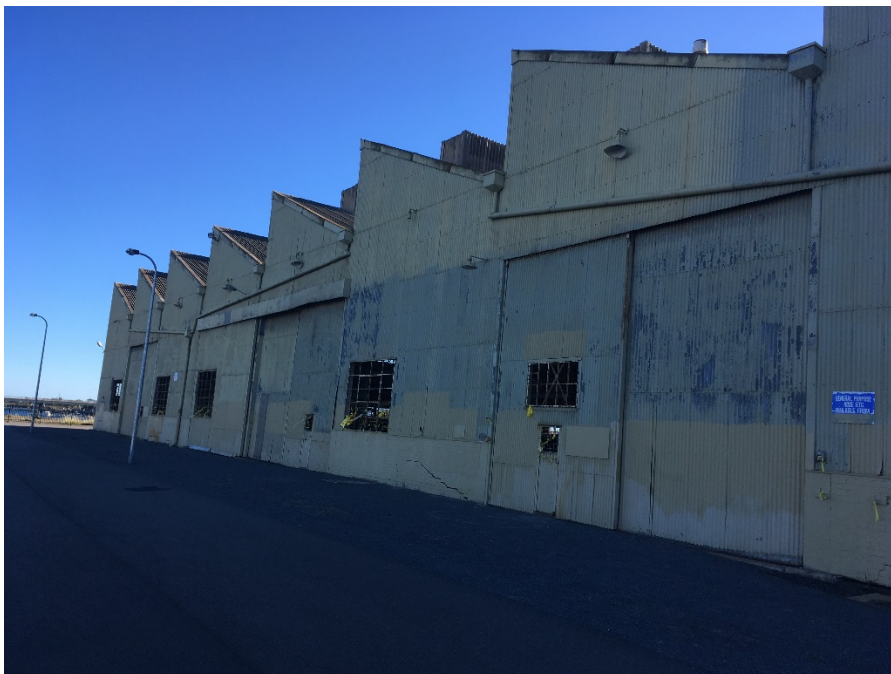
Shed 26 showing the eastern elevation, note the hoods on the ridgeline of each sawtooth.
