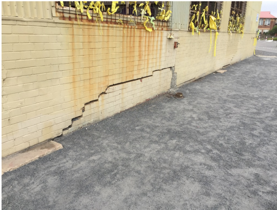
Shed 26 showing cracking on the eastern façade.
