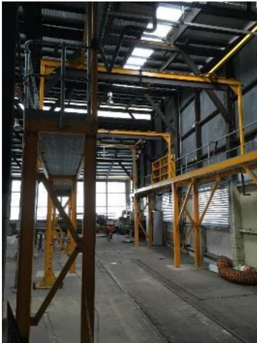
Inside the roundhouse showing the original and modern gantries.
