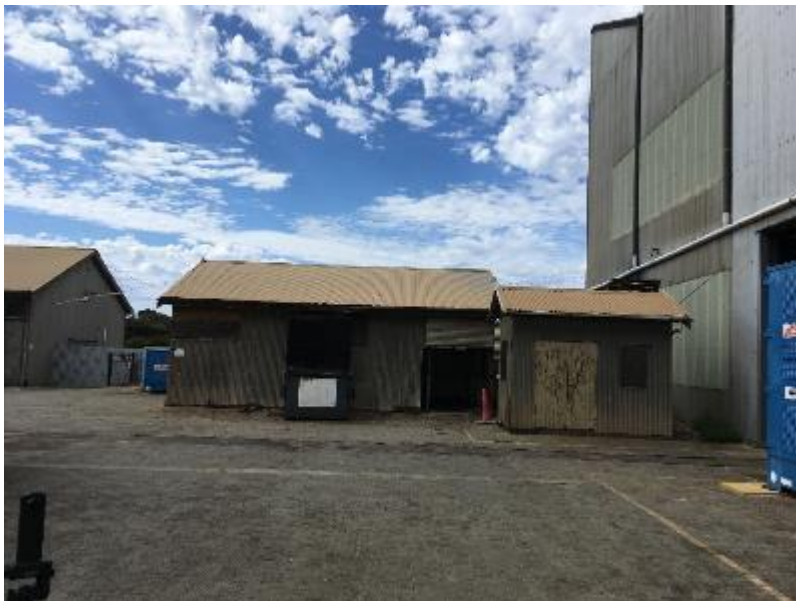
Shed adjacent to the locomotive workshop.
