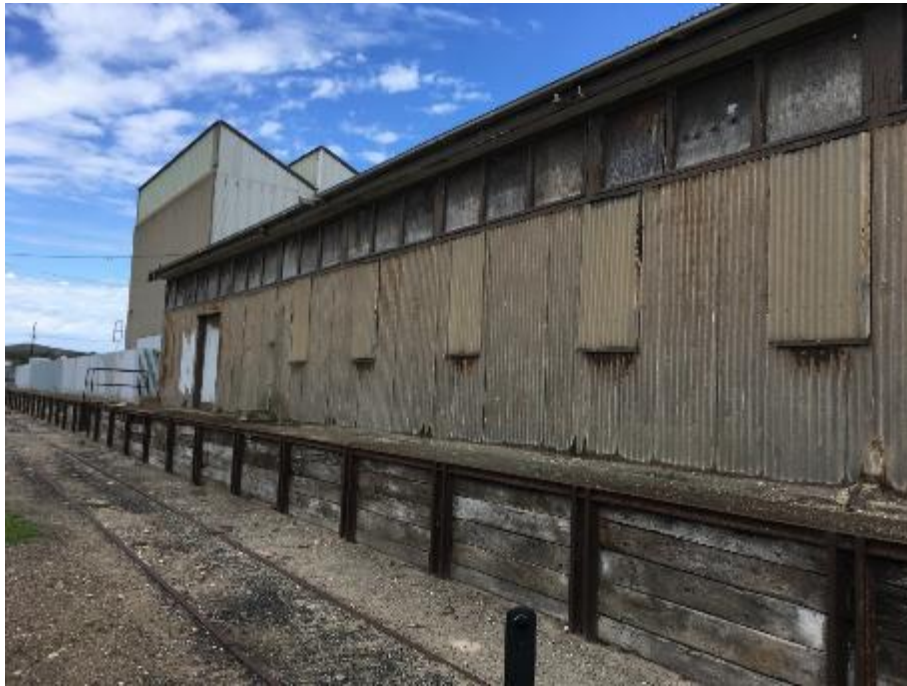
View of the divisional store and adjacent siding.
