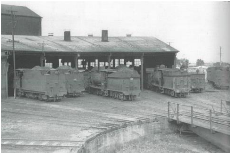
Roundhouse at Port Lincoln Locomotive Depot and Workshops, images taken in 1959, note the multi-pane windows and open front.
