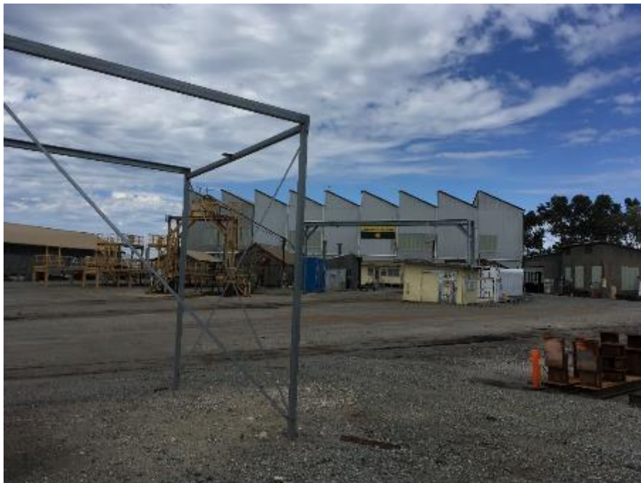
View of the workshops showing the relationship between the locomotive workshop and the roundhouse and running car shed, and the range of structures on site.
