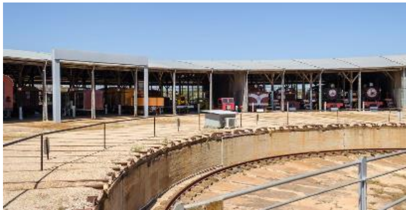
Peterborough Roundhouse as it appeared in 2018, ongoing repairs include replacement of the damaged and lost panes of glass due to wind damage.
