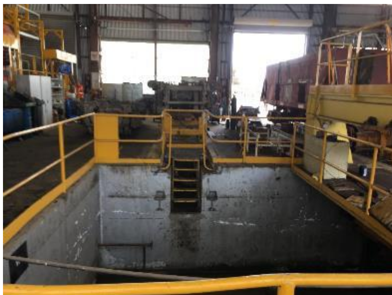
Inspection pit inside the locomotive workshop.
