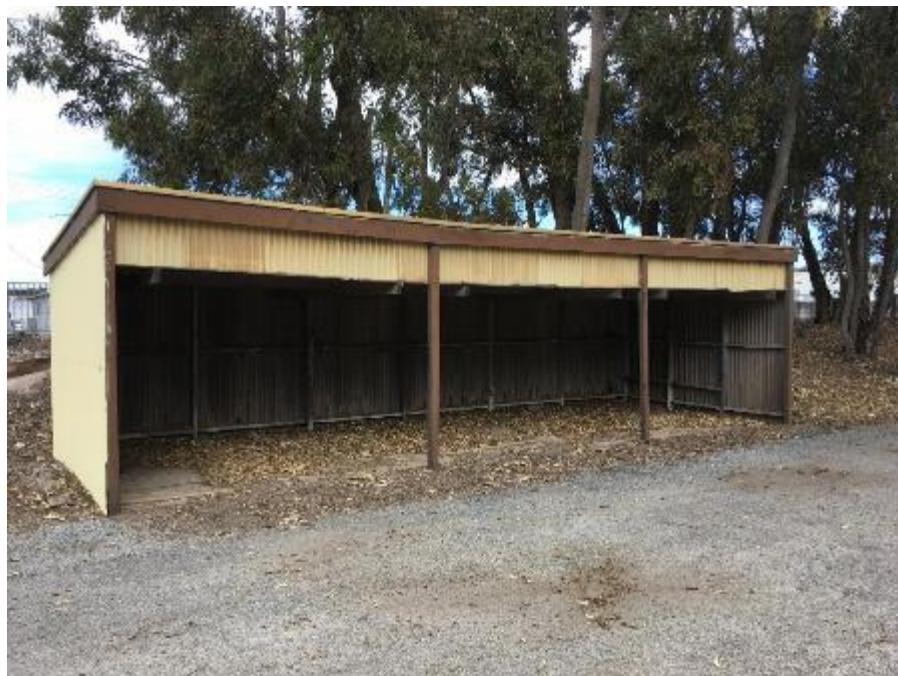
Shed with timber sleeper floor, possibly a bike shed.
