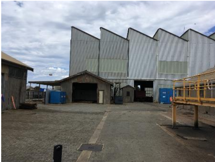
View of shed in the yard.
