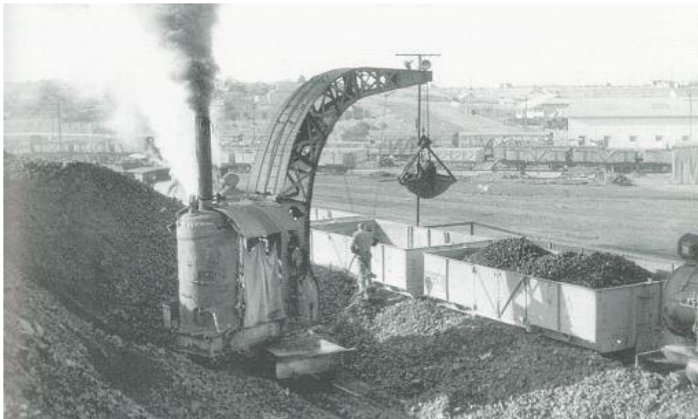
Cowan & Sheldon coaling crane in the coal dump at the Port Lincoln Locomotive Depot and Workshops, image taken in 1965.
