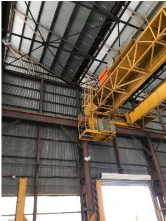
Locomotive workshop showing the crane gantry and newer crane addition.
