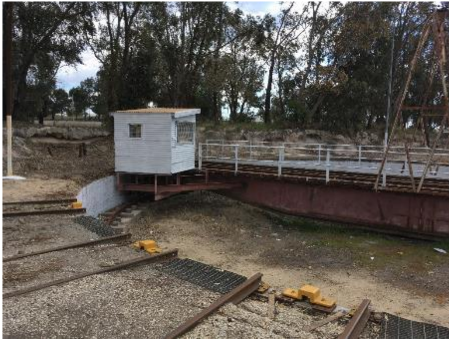
Turntable, showing the cabin and gantry.
