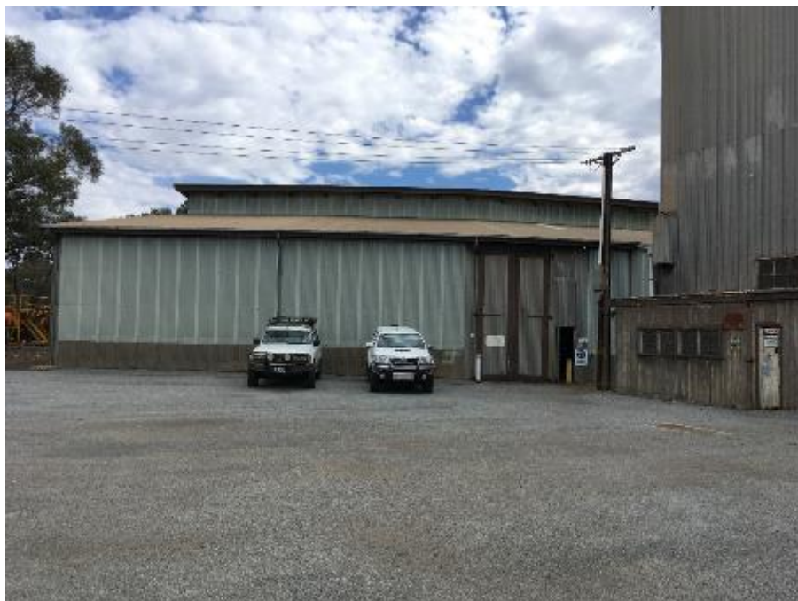
View of the exterior of the roundhouse, note the replacement of the windows with polycarbonate sheeting.
