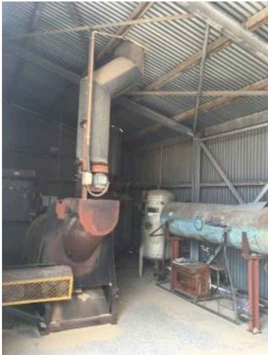
Example of machinery inside shed in the yard.
