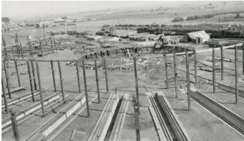
Peterborough Roundhouse under construction mid-1920s
