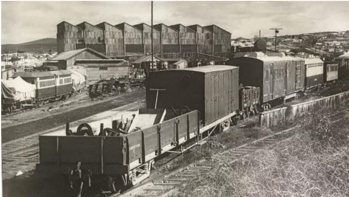
View of the Port Lincoln Locomotive Depot and Workshops looking towards the locomotive workshop, note the variety of sheds in the yard, image taken in 1967.
