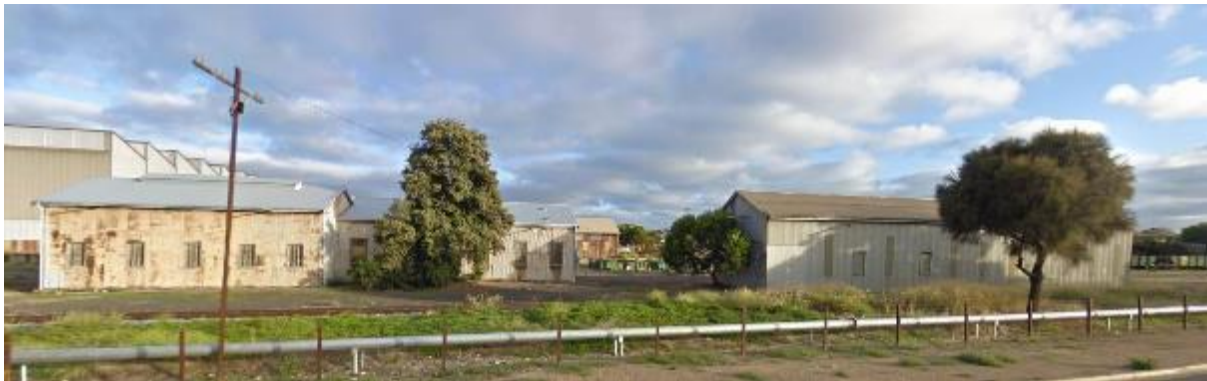
Painters' (left) and Carpenters' (right) workshops (now demolished).
