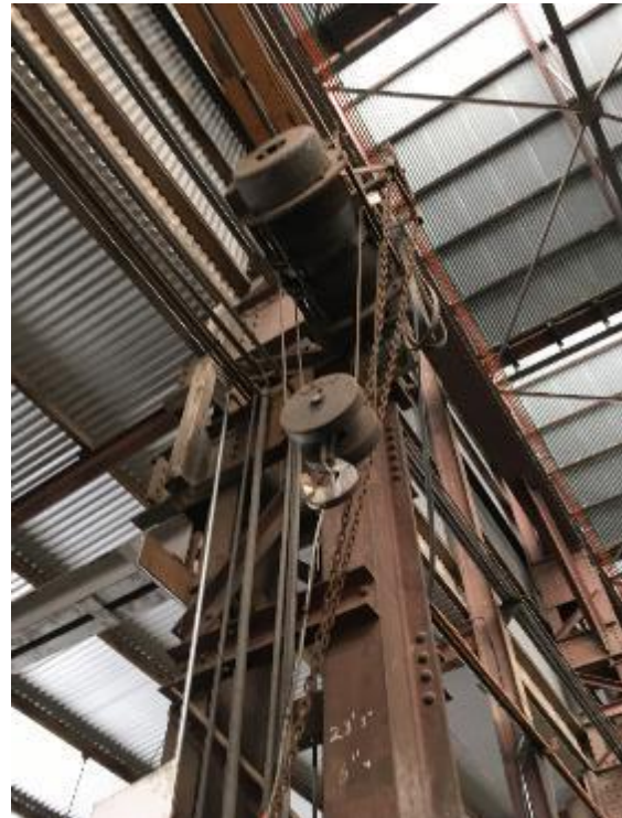
Locomotive workshop showing an example of the older equipment still inside the building.
