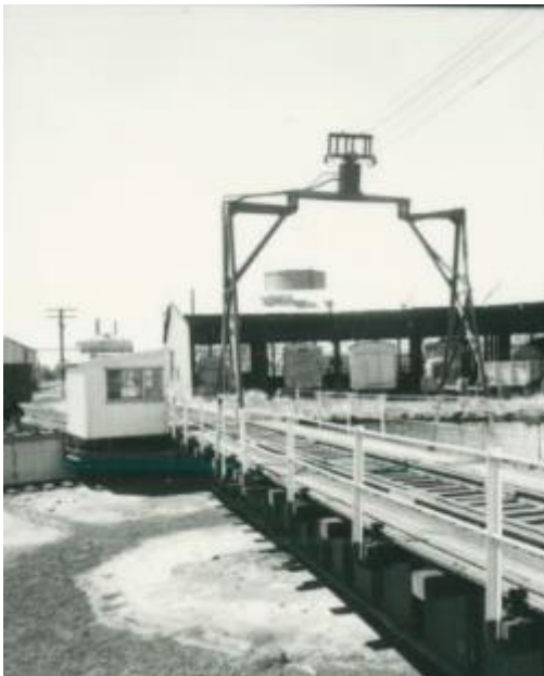
Peterborough Roundhouse and Turntable as it appeared in 1984 prior to State heritage listing.
