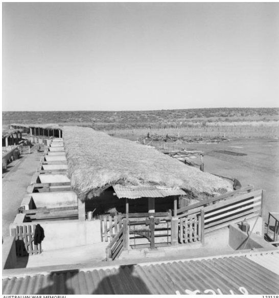
View of the breeding pens (subject of this assessment) from the roof of the boiler house, note the loading ramp.
