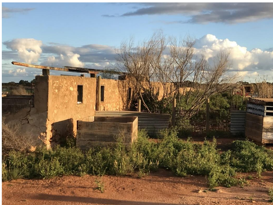
Detail of the wall western elevation, note cracking and loss of render, the fencing is a later replacement
