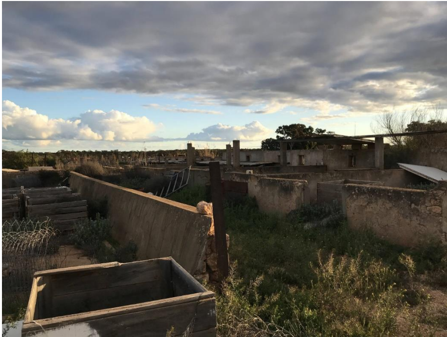
Internal wall of the eastern pens, timber fencing to complete each pen has been removed
