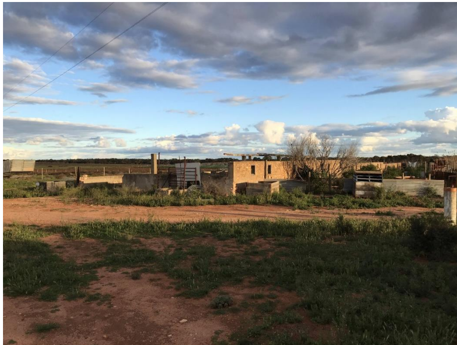
Northern elevation of the piggery breeding pens
