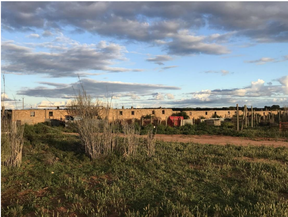
Higher outer (western) wall showing window openings
