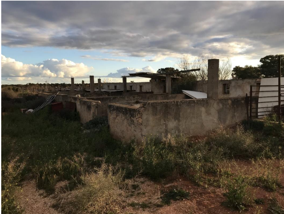
Pens on the western side of the structure
