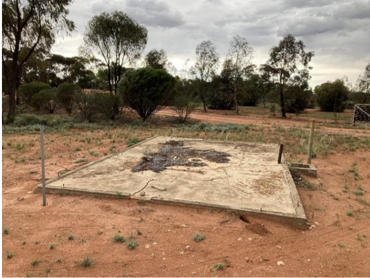
Concrete slab for the Mortuary, Loveday Internment Camp Complex, note central drainage point and additional drain to side of slab.
