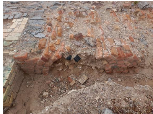
Calciner 1 cooling vault Source: DEW Files 1 March 2022
