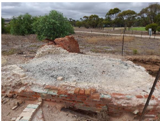
Refractory sand hearth of Smelter B with remains of elliptical firebrick walls Source: DEW Files 1 March 2022
