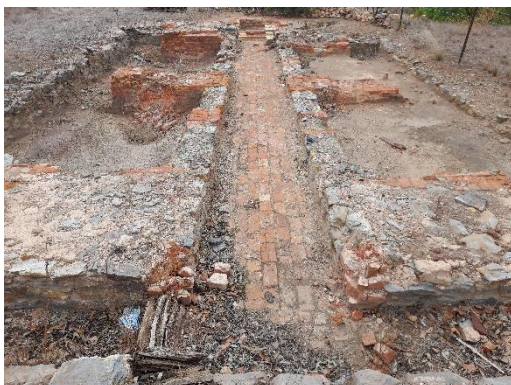
Calciner 2 paved central channel
