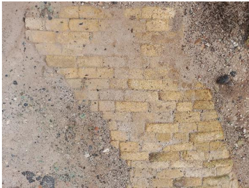
Paved firebrick working floor
