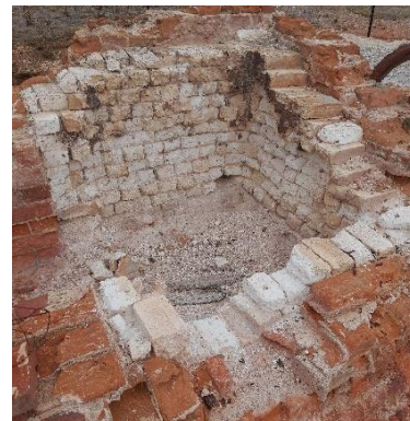
Chimney of Smelter B showing firebrick core
