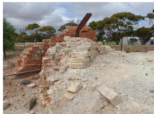
Hearth of Smelter B showing coursed firebricks Source: DEW Files 1 March 2022
