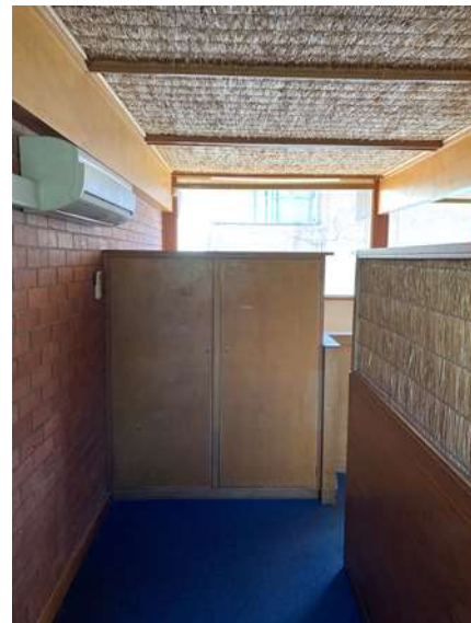
Filing space in the drawing room, the top of the partition was originally glass, note addition of air conditioning unit.
