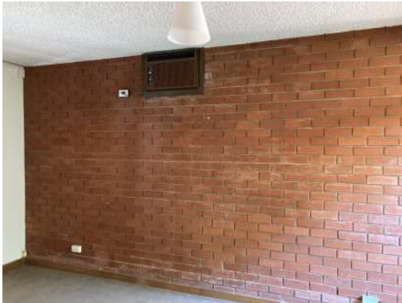
Principal's Office showing face-brick wall and addition of air conditioning unit.
