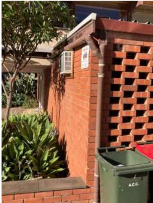
Office Building 2021, note the addition of guttering and downpipes, insertion of air conditioning unit through the wall.
