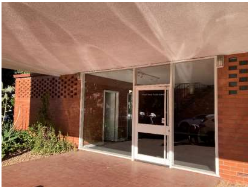
Entrance, note the loss of name plate and modifications to door, painting of timber, addition of lights.
