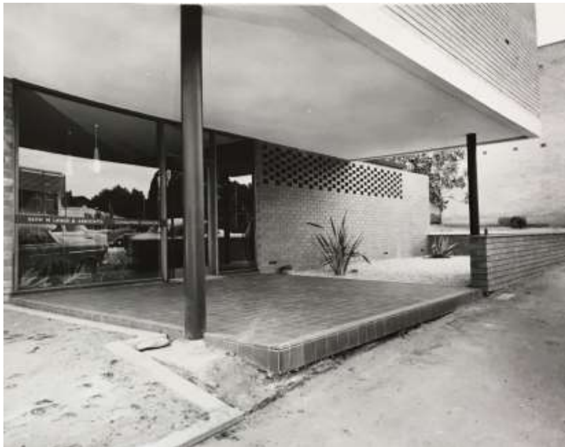
Office Building 1965, eastern elevation, note perforated brickwork, tile, name plate to glass.
