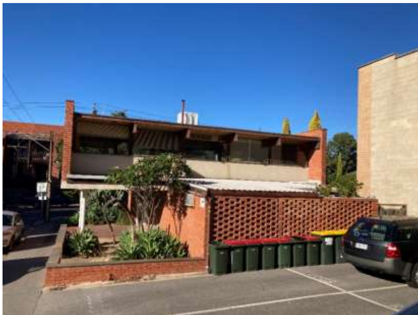
Northern elevation, note change to perforated-brick-wall, extended roof into courtyard, metal roofing, addition of fascia to guttering.
