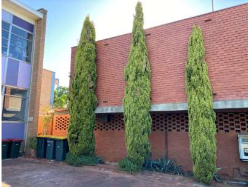
Western elevation, note the addition of the air conditioning unit through the wall.
