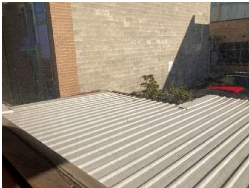
Roof to north showing addition of metal cladding.
