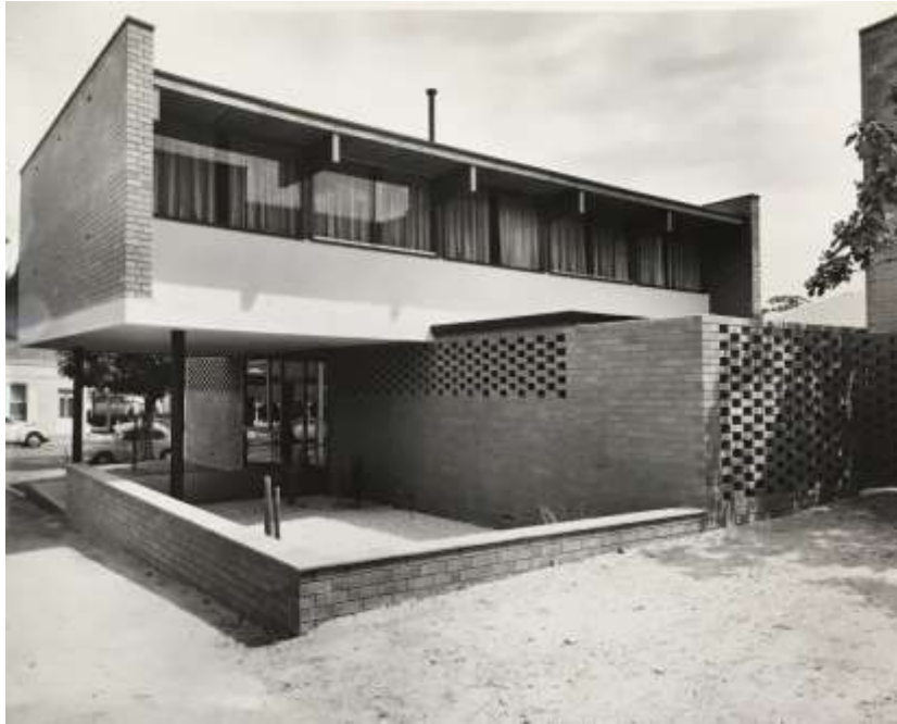
Office Building 1965, northern elevation, note garden & brickwork.
