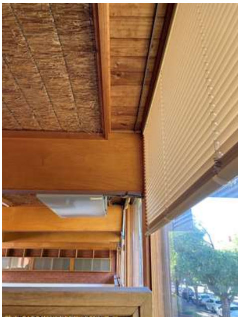
Ceiling to drawing room showing the timber framed Solomit® straw panels, and channel created by the framing to accommodate the lighting.
