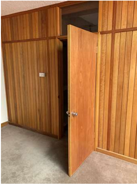
Timber partition wall to create new office space.
