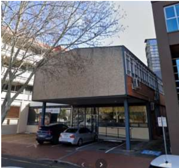
Metropolitan Milk Board Building, Hutt Street Adelaide, 1962, Hassell & McConnell
