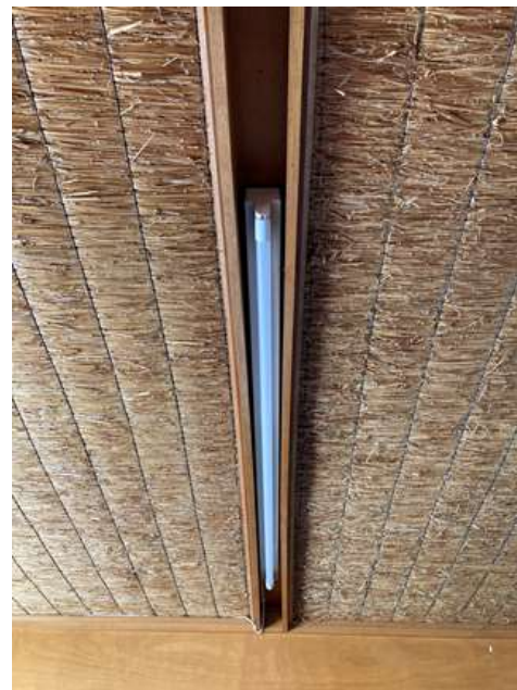
Ceiling to drawing room showing the timber framed Solomit® straw panels, and channel created by the framing to accommodate the lighting.
