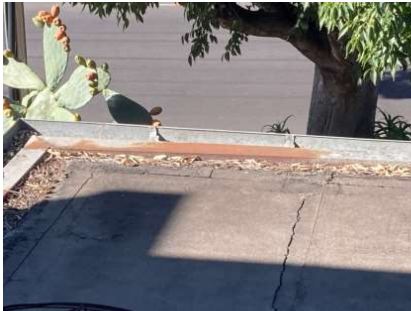
View of roof to south showing the original flat roof, with formed gutters (filled with leaves) and additional guttering abutted to it.
