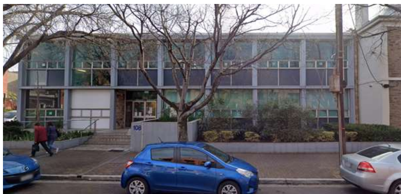
Bradford Insulation, Kermode St, Adelaide, Caradoc Ashton Woodhead Hall McDonald Shaw
