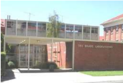
Bragg Laboratories 1962 Example of International Style and Miesian architecture
