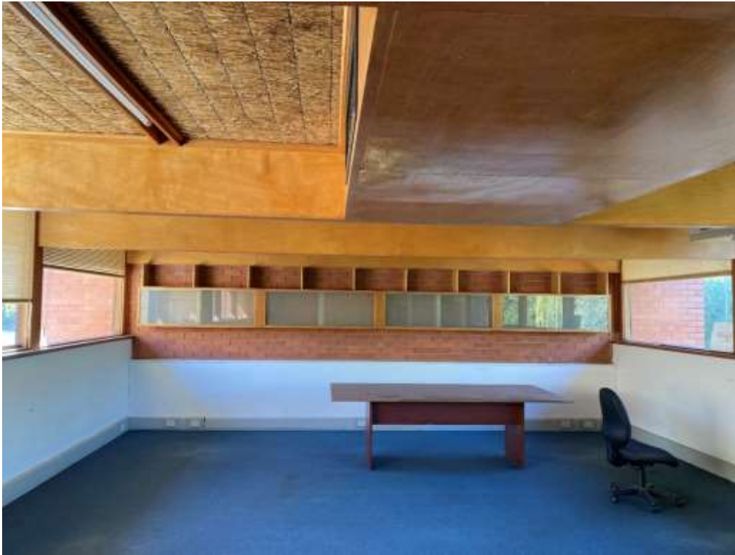
Drawing Room, showing the bespoke wall-mounted cupboard, Solomit® straw ceiling panels, plywood boxed beams, plywood-clad air conditioning ductwork. Note the new carpet, loss of low cupboard and desks.
