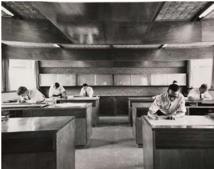
Office Building 1965, drawing room, note the linoleum floor, bespoke low and wall-mounted cupboards, and desks.
