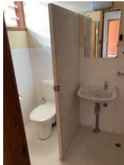
Example of bathroom, showing terrazzo partition wall, tile and original sink and towel rail.
