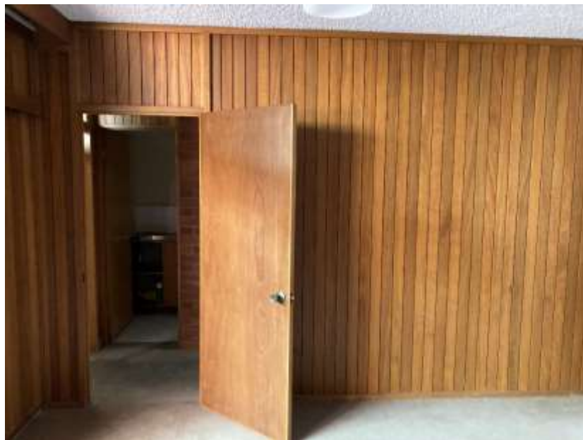
Principal's Office, timber partition wall added to create corridor.
