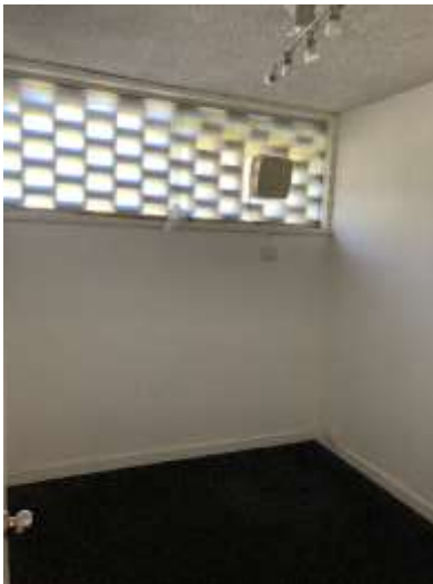
Printing room, note addition of exhaust fan through glazing and perforated brick wall.
