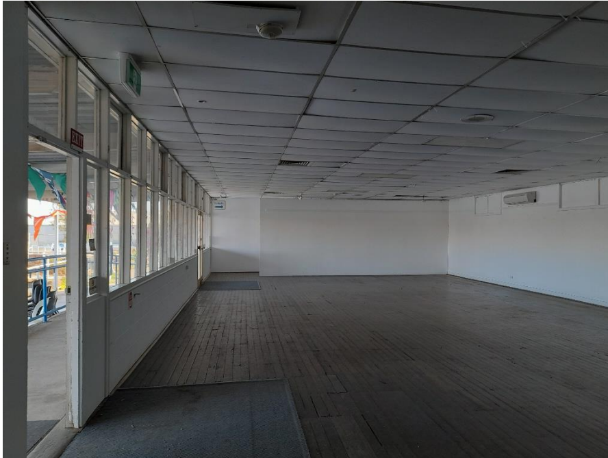
Former Port Adelaide Sailing Club premises, interior function space
