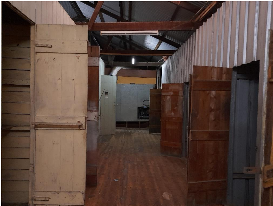
Former Port Adelaide Sailing Club premises, interior showing storage lockers
