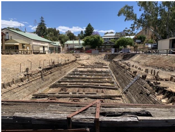
Former 'Randell' Dry Dock, 1873, Mannum (SHP 10282)
