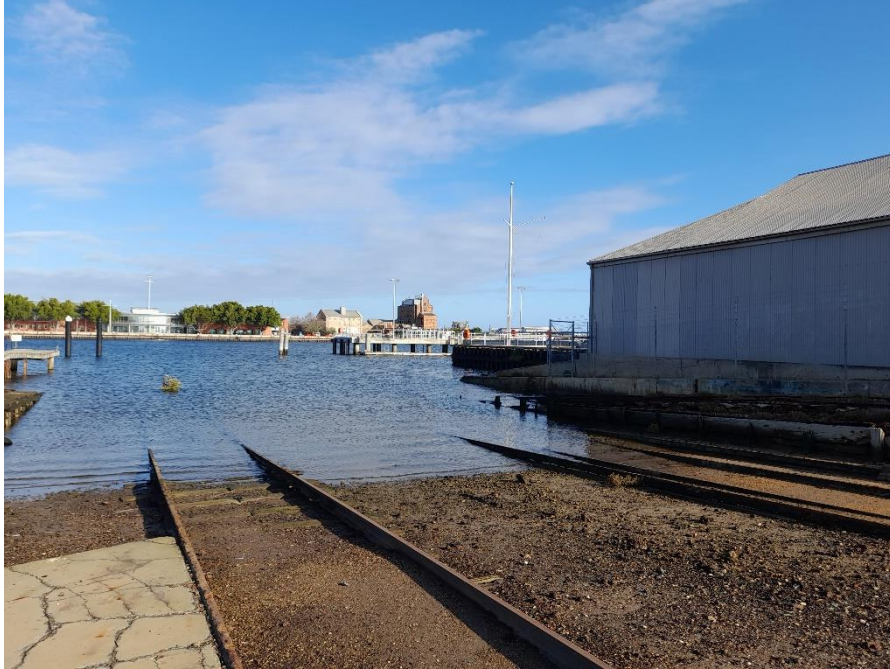
Jenkins Street Slips Precinct, slips in vicinity of former Searles Boatyard
