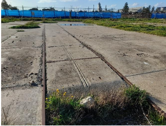
Detail of slipway showing floor slabs
