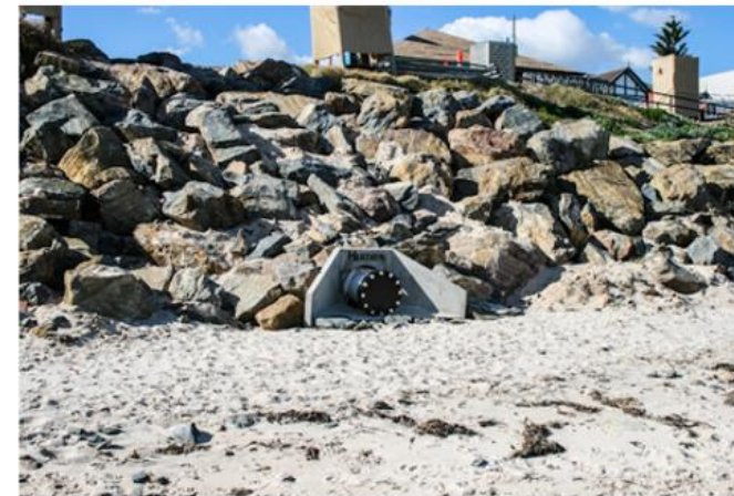
Sand pumping discharge pipe (DEW)
