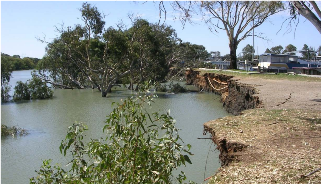
Figure 14: Riverbank collapse at Long Island Marina, Murray Bridge
