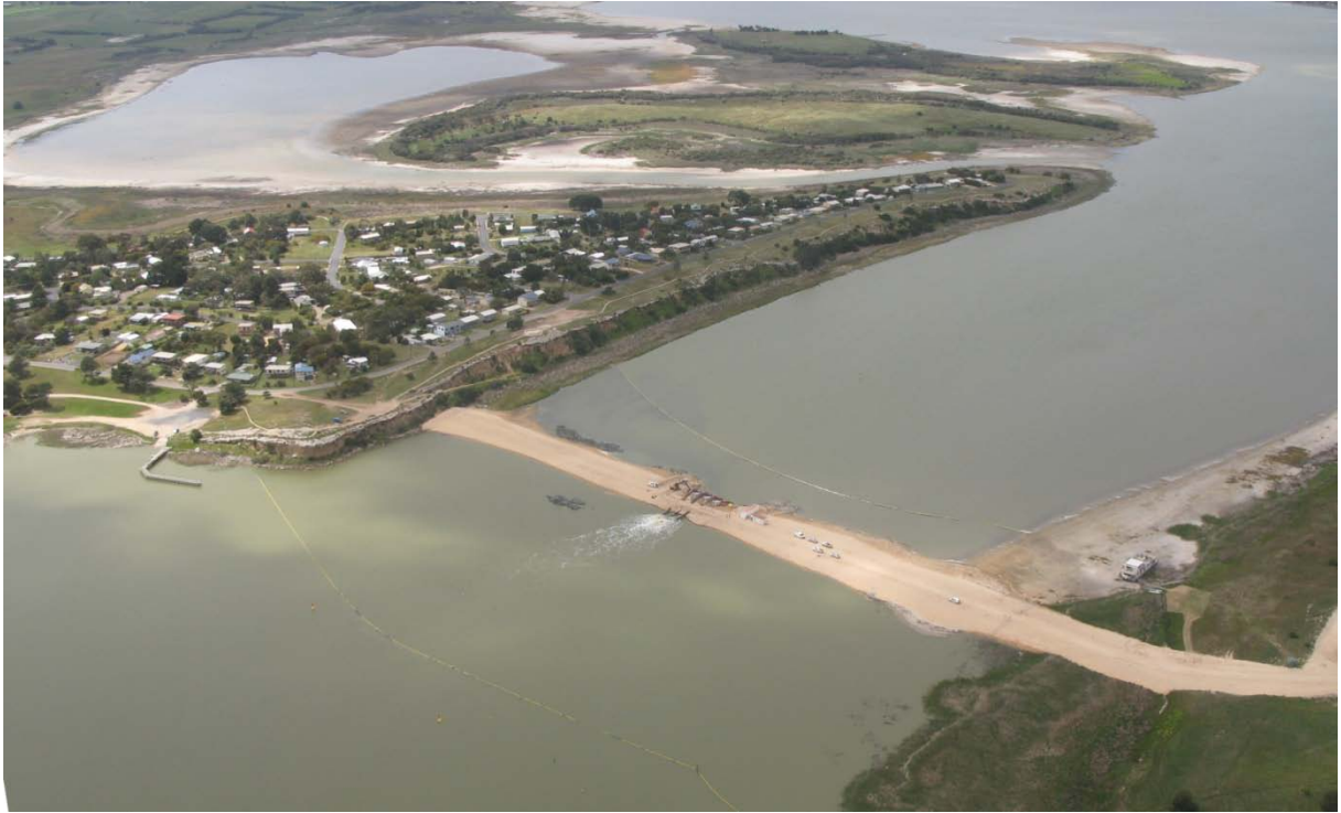
Figure 5: Temporary regulator at Clayton, October 2009
