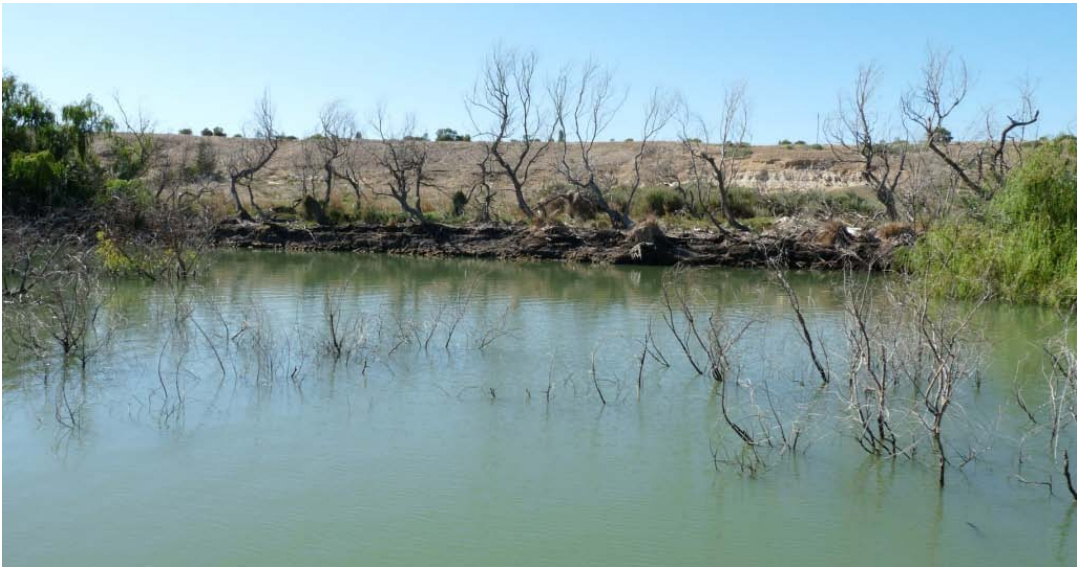
Figure 13: Riverbank collapse at Fred’s Landing near Tailern Bend
