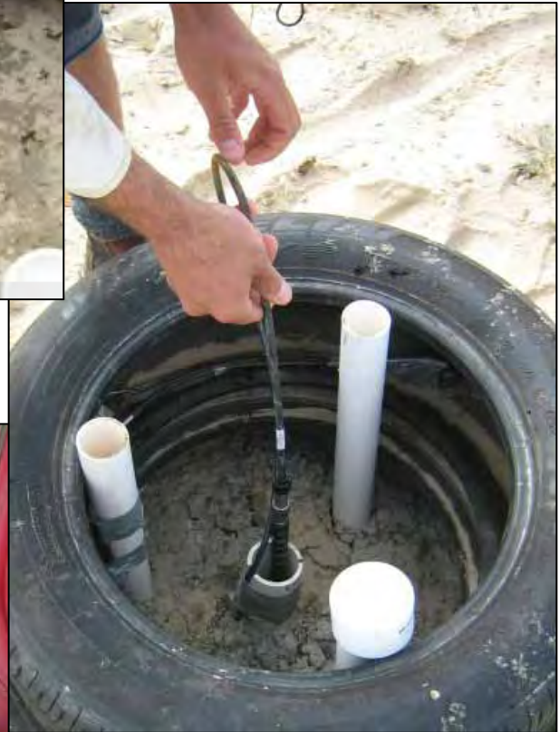
Plates 14-15. Installation of groundwater (piezometric) levels sensors.
