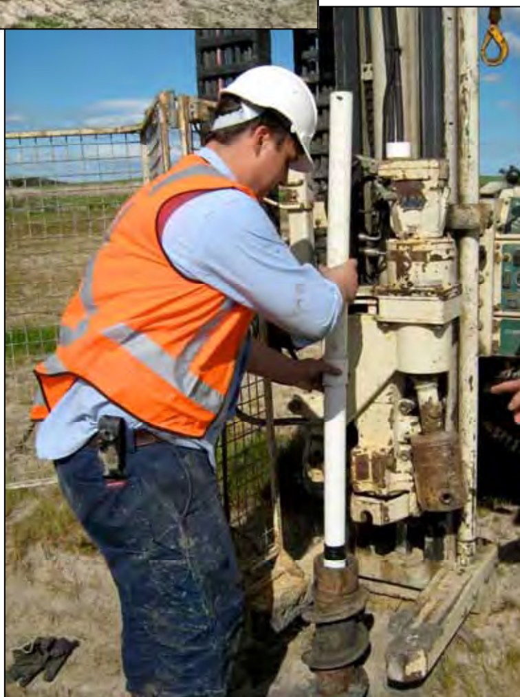
Plate 13. Hollow auger system used for piezometer installation. After inserting the piezometer to the required depth, the auger hole was backfilled with clean sand around the screened section and then capped with bentonite, whilst progressively removing the hollow auger rods.
