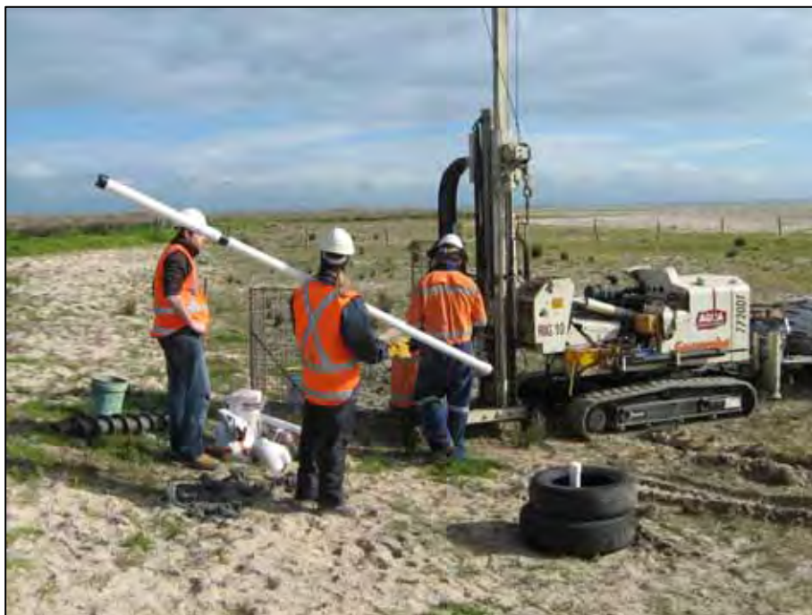
Plate 12. Piezometer installation at Campbell Park, Lake Albert.
