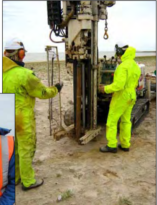
Plate 3. Double-tube push tube sampling conducted using a 7720DT Geoprobe drill rig.
