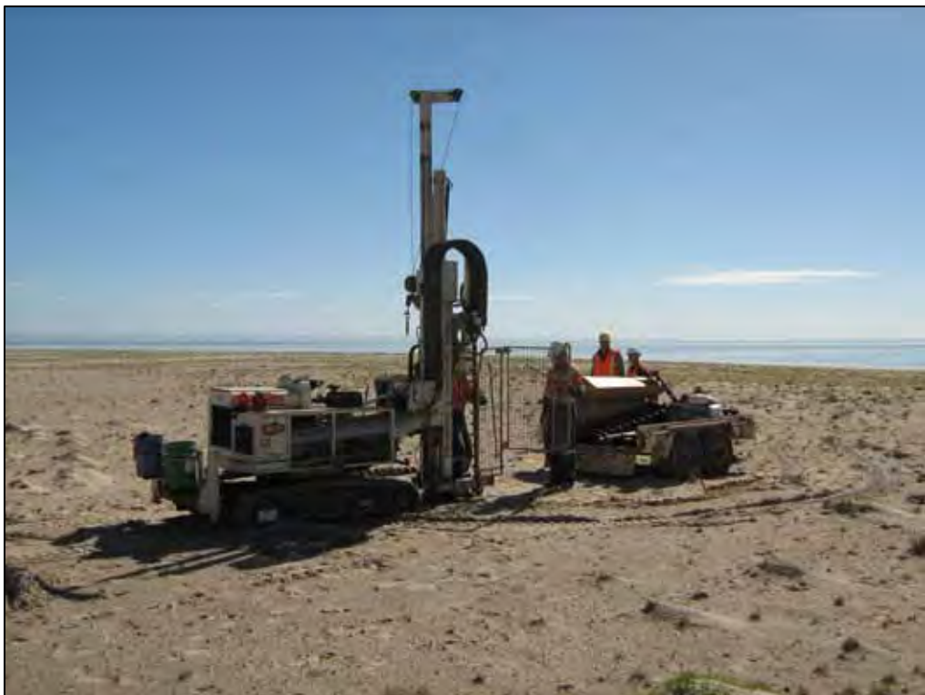
Plates 10-11. Geoprobe 7720DT drill rig used for sediment sampling and piezometer installation at Point Sturt (pictured), Campbell Park and Windmill locations.
