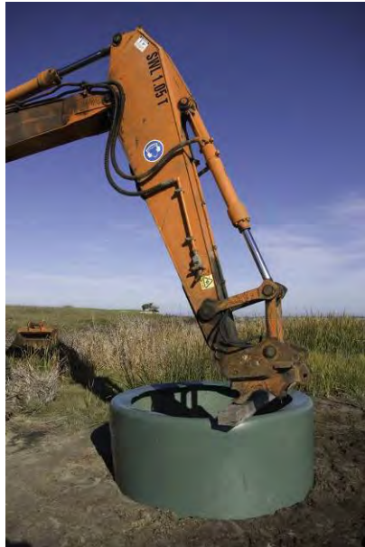
Figure 4 Tank installation at the Boggy Ck. site
