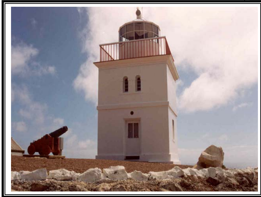
Cape Borda Lighthouse Courtesy Coastal Protection Branch.
