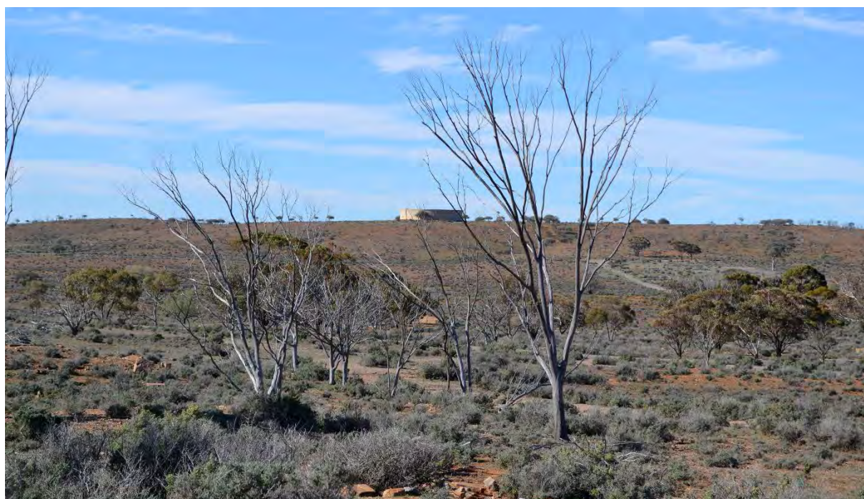
2million Gallon Tank on hilltop, 2016
