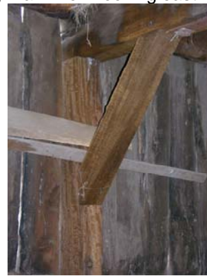
Detail of Slab Barn No 1 interior
