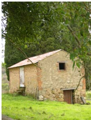
Stone outbuilding looking north from track
