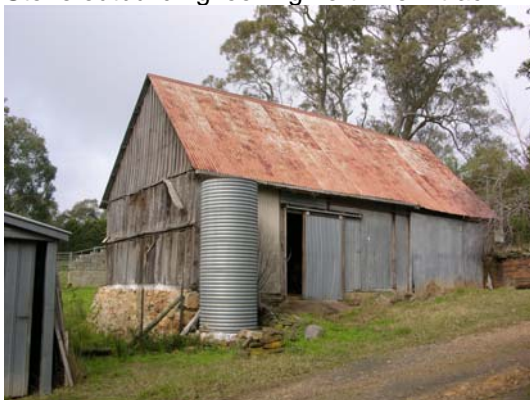
Slab Barn No 1 (looking south)
