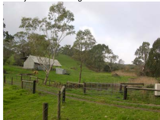
Slab /cgi Barn No 2 looking east from track
