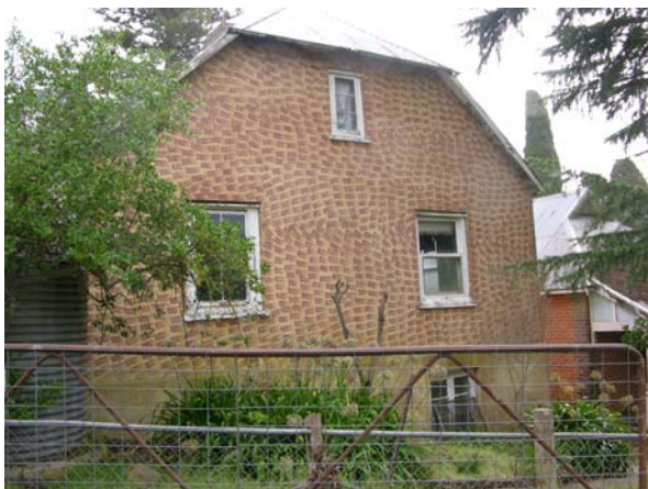
Eastern façade looking west from track
