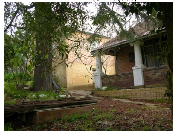
Twentieth Century addition looking south west towards rear of main house
