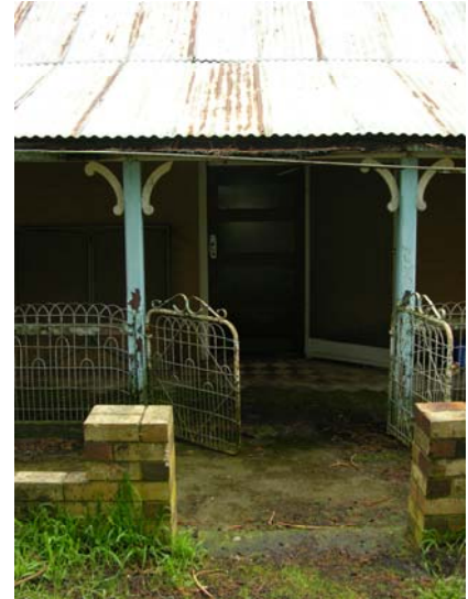
Front door of 1840s house (SW façade)
