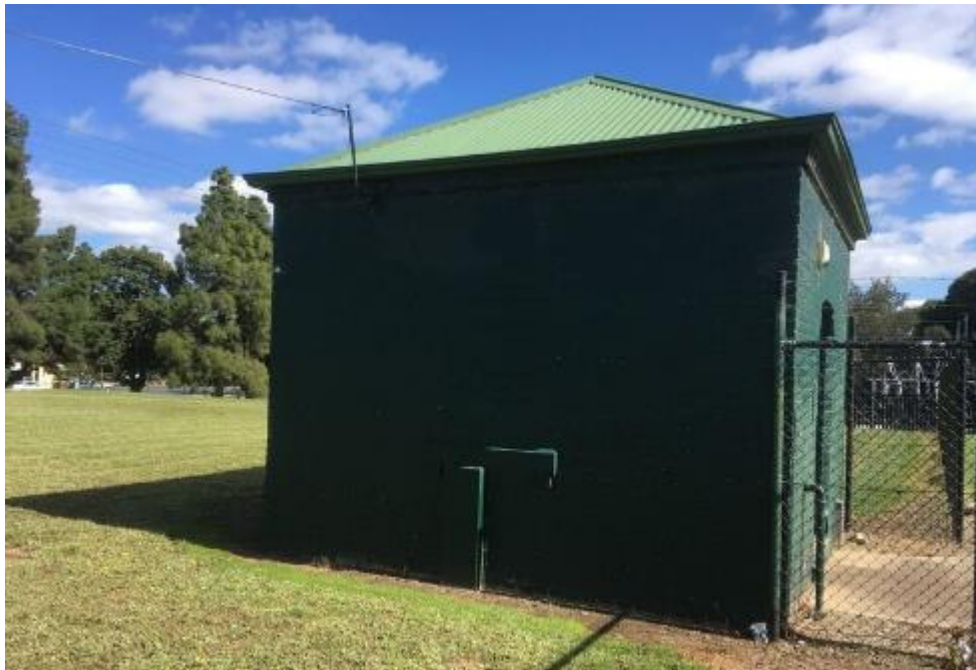
North Adelaide Service Reservoir pump-house
