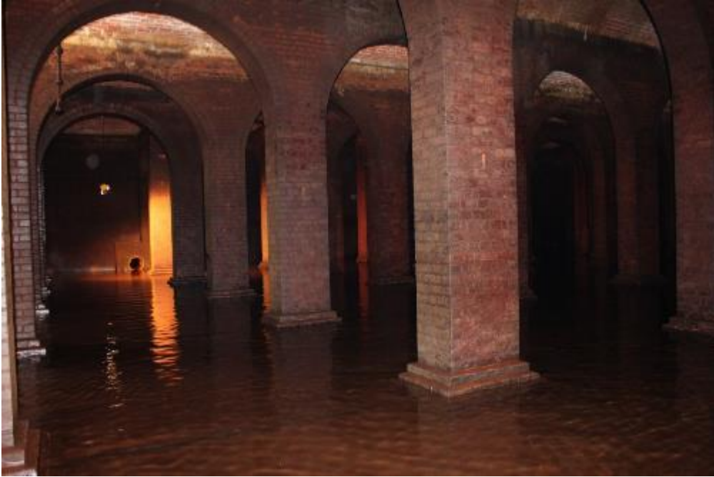
North Adelaide Service Reservoir interior (courtesy SA Water)
