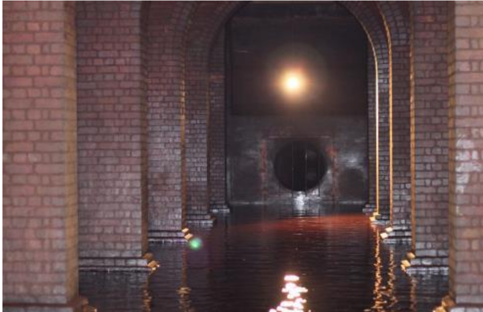
North Adelaide Service Reservoir interior (courtesy SA Water)
