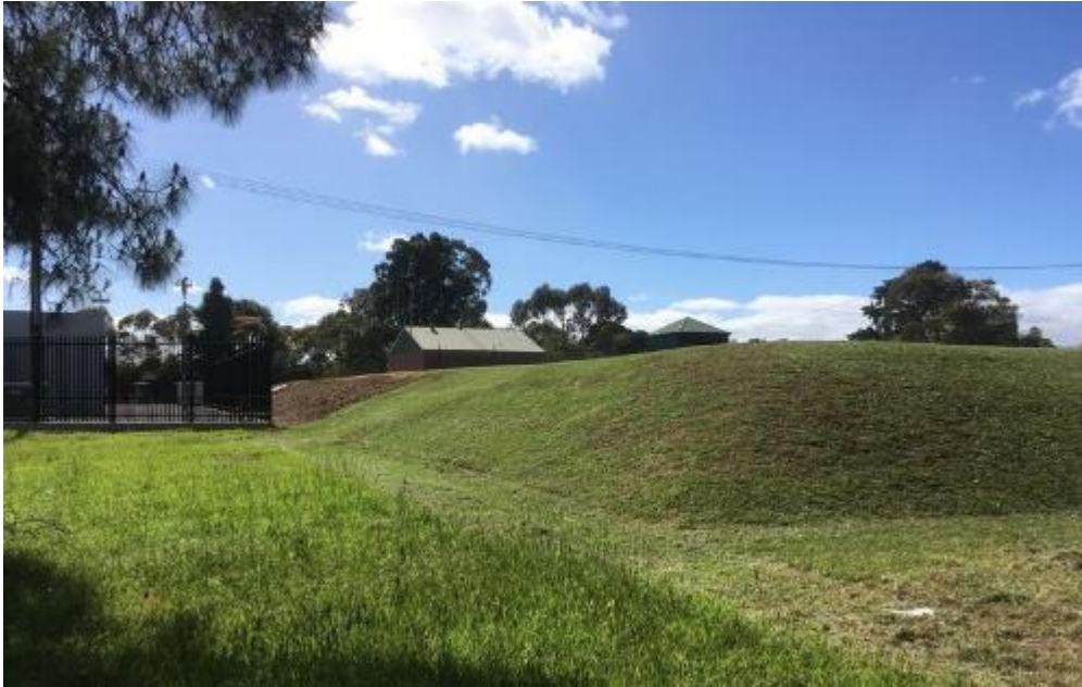
North Adelaide Service Reservoir mound
