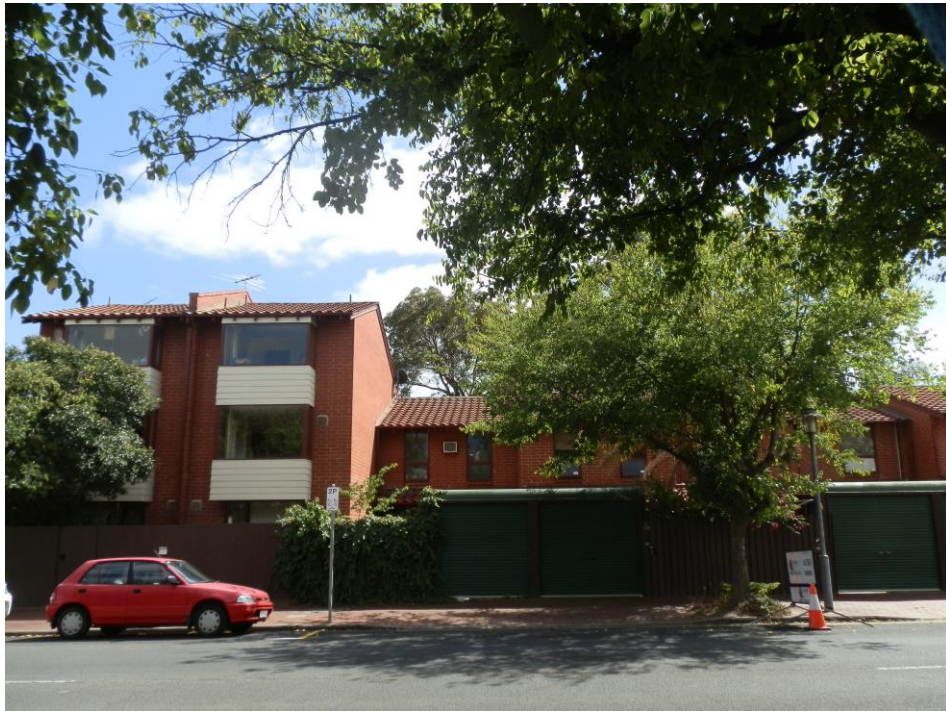
Manitoba Housing Complex, Carrington Street, Adelaide – Two and three storey units on Carrington Street (looking north) (March 2014)
