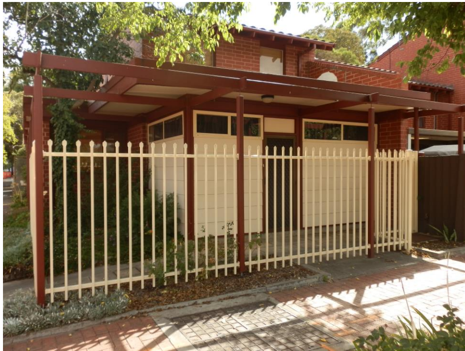
Manitoba Housing Complex, Carrington Street, Adelaide – Former barber’s shop, corner of Carrington Street and Regent Street North (looking north) (March 2014)
