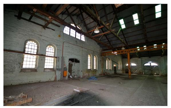
Old Bulk Store – Interior – note original central metal web truss and support columns
