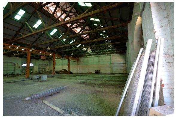
Old Bulk Store – Interior – note later steel/reinforced concrete infill wall Department of Environment, Water and Natural Resources
