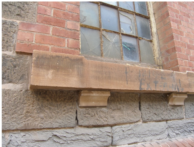
Old Bulk Store – Detail showing window sill
