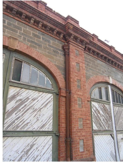
Old Bulk Store – Detail showing decorative elements of the building – note parapet
