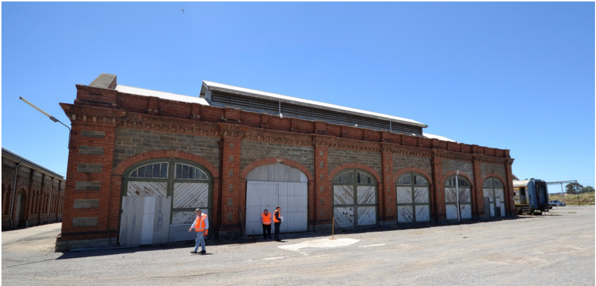
Old Bulk Store – View from south
