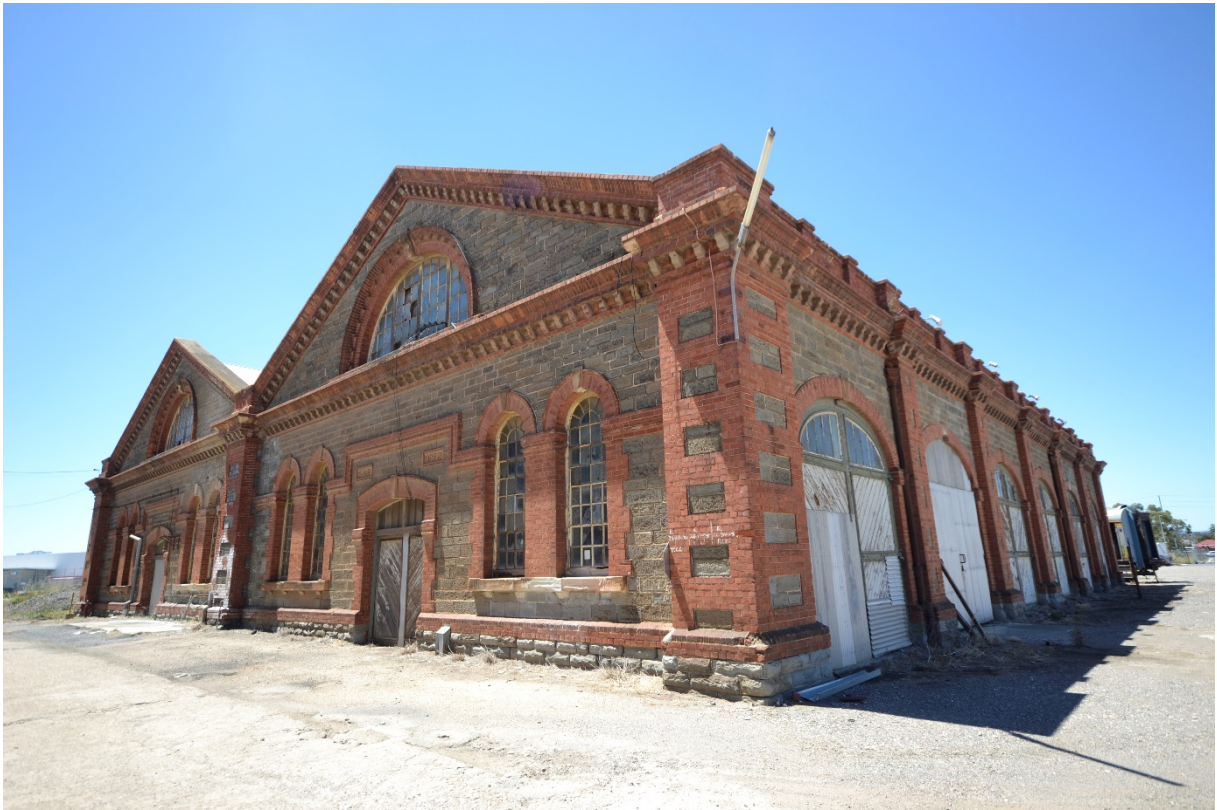
Old Bulk Store – View from south-west corner
