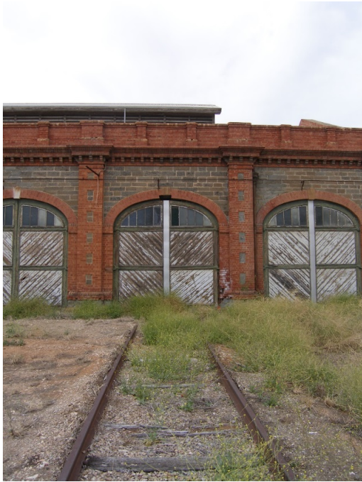
Old Bulk Store – View from north
