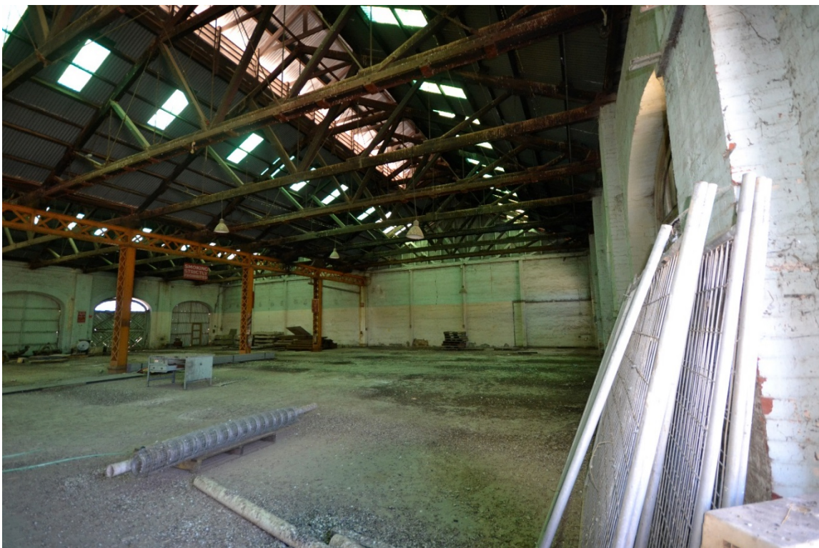
Old Bulk Store – Interior – note later steel/reinforced concrete infill wall
