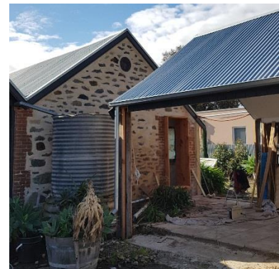
Building 2. Open-ended kitchen area. July 2017
