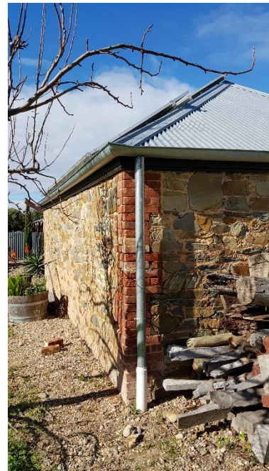
Building 1. North elevation. Note hipped roof. July 2017 Source: DEW
