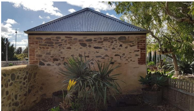
Building 2. South elevation. Note bluestone and redbrick construction at the top of the wall with render below. July 2017.
