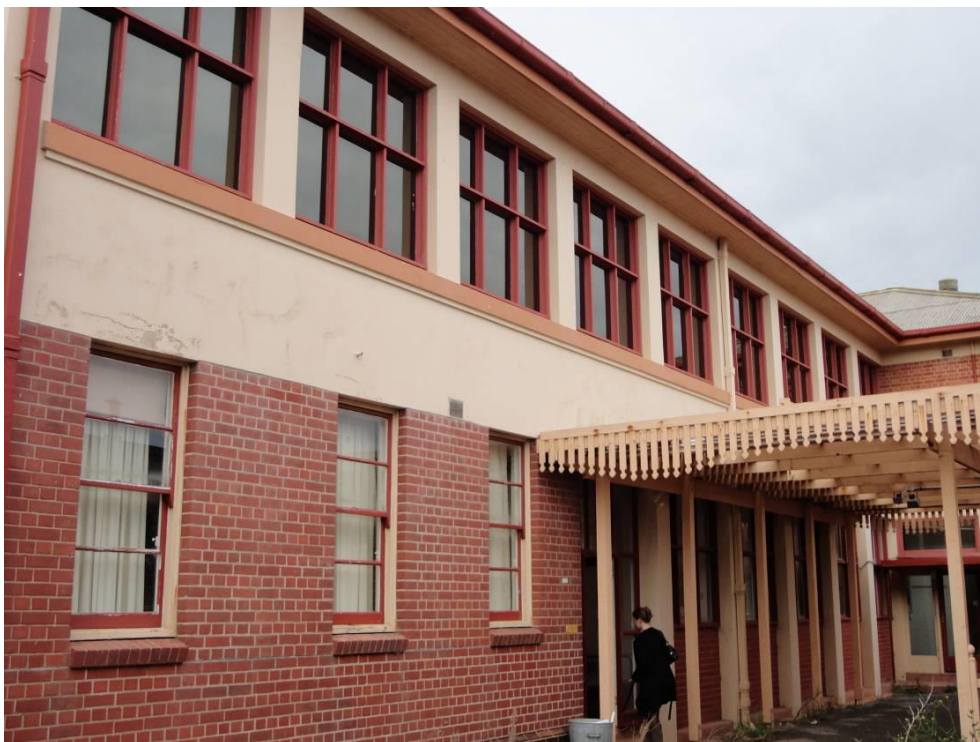
West Façade of Barracks Building [note later enclosed upper balcony & ground level verandah] ( Grieve Gillett 2014 )
