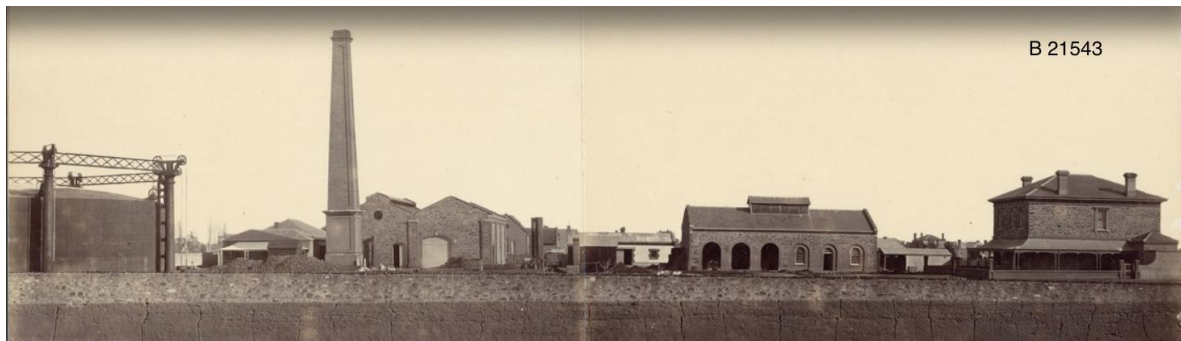
Brompton Gasworks attributed to Captain Sweet, c1870 (B21543, courtesy of State Library of SA). View is from NE, possibly from Second St – note pug hole in foreground. [Other texts note this image was taken from the railway line – this is incorrect.]
