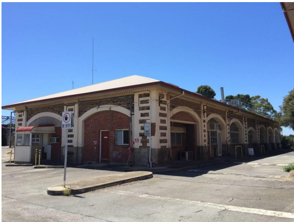
Former SAGASCO Gasworks, Brompton – Building B22 (Former Purifying House), from SE end (2015)
