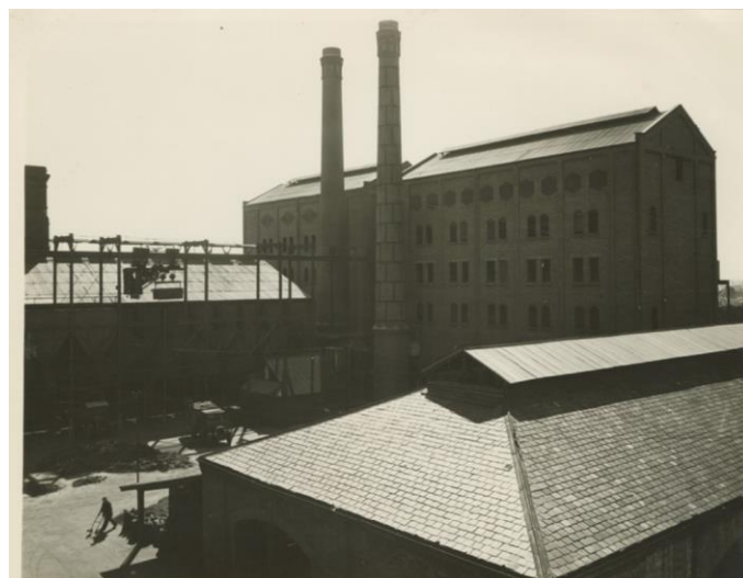
Shows now demolished vertical retort houses, along with the roof of B22 (Purifying House), with slated roof (BRG 350/34/1/2/1, Courtesy of the State Library of SA)
