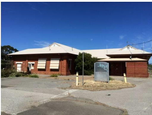
Former SAGASCO Gasworks, Brompton – Building B29 (Former Administration Building), view from NW side (2015)
