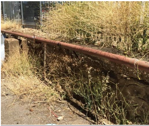
Former SAGASCO Gasworks, Brompton – Sundry platform walls, view from railway line (2015)
