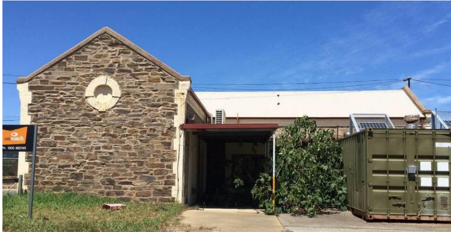
Former SAGASCO Gasworks, Brompton – Building B27 (Former Chemistry Laboratory), view from NW side (2015)
