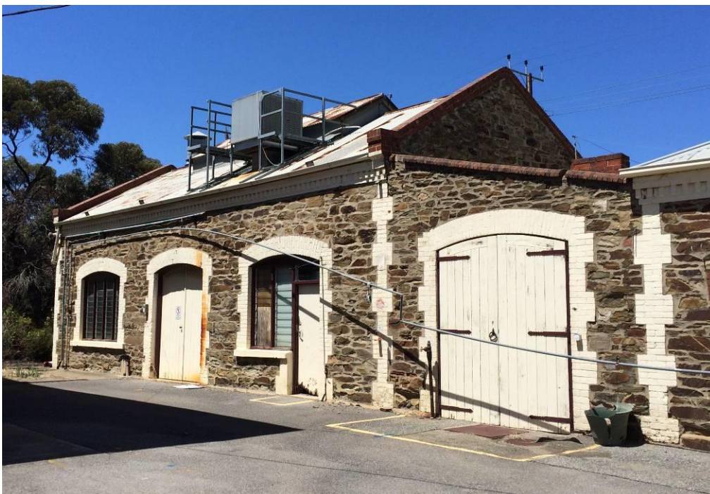
Former SAGASCO Gasworks, Brompton – Building B106 (Former Carpenter's Workshop), view from NW side (2015)
