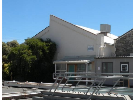
Former SAGASCO Gasworks, Brompton – Building B18 (Workshop/ Store), view from SE side (2015)
