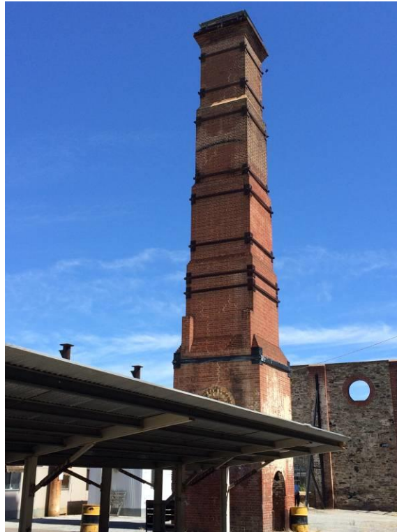
Former SAGASCO Gasworks, Brompton – Building SHP 3 (Horizontal Retort House 4 Chimney), from NE end (2015)
