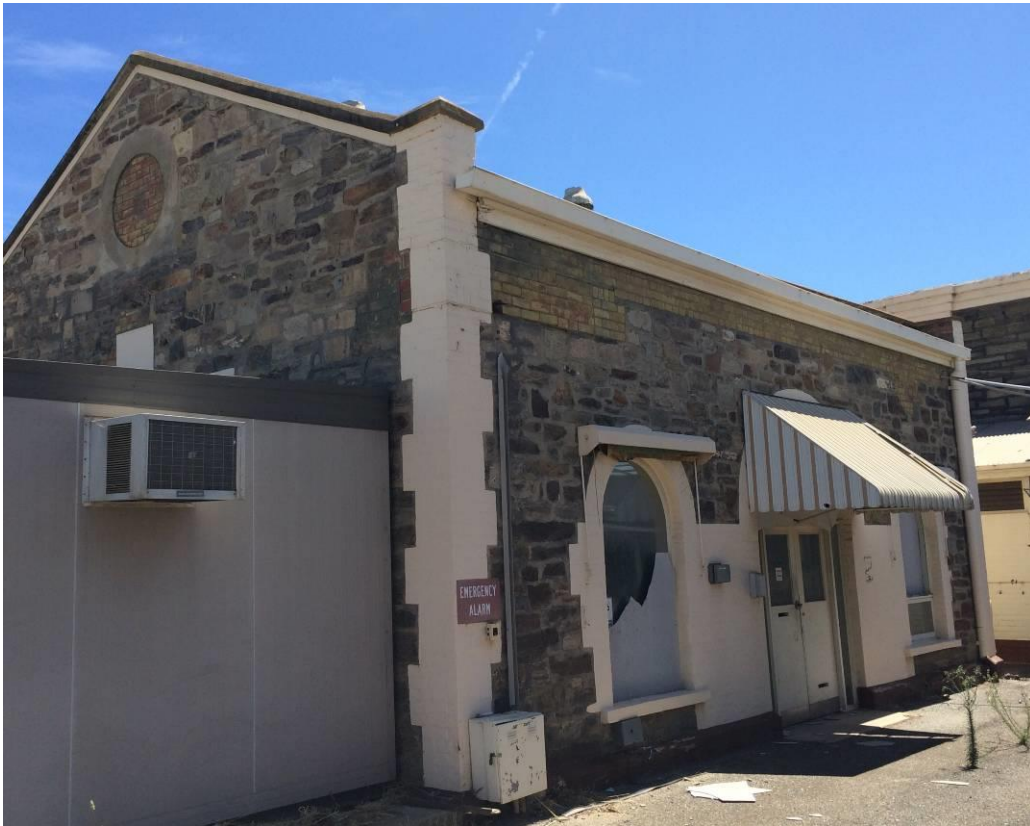
Former SAGASCO Gasworks, Brompton – Building B18 (Former Boiler House), view from NE end (2015)
