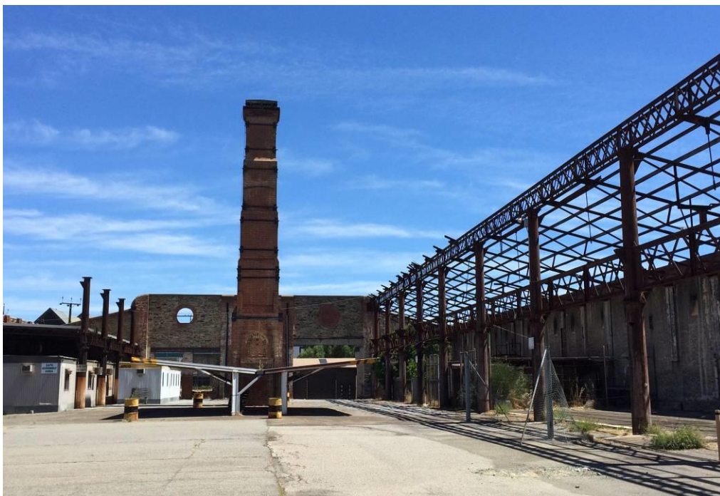
Former SAGASCO Gasworks, Brompton - Building SHP2 (Horizontal Retort House 4) from NE end (2015)
