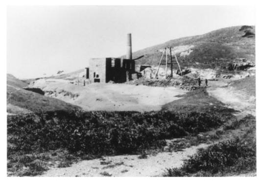
Prince Alfred Copper Mine, 1915 - View is toward the northeast. (*Mining Review* No. 25). [The Engine Shaft headframe is still standing. Note the large quantity of tailings in this photograph before they were removed for leaching.]
