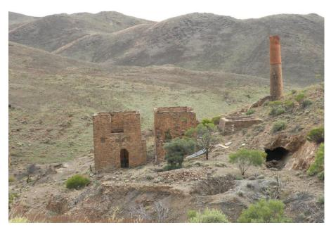
Prince Alfred Copper Mine Precinct, via Cradock - View to north [Crusher house, engine house and water tanks to supply boilers; chimney and flue at rear; two shafts in mid-ground and open stope at right.]
