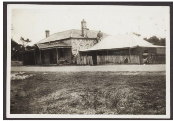
The Rumbelow family residence in Franklin Parade, Yilki, c 1880. The original home on the right was a wooden structure referred to by the family as the 'Crystal Palace'; the stone house on the left is 'Yeltanna'. Source State Library South Australia B-27477
