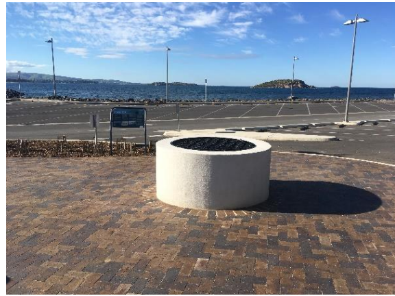
Site works complete June 2019 Source DEW
