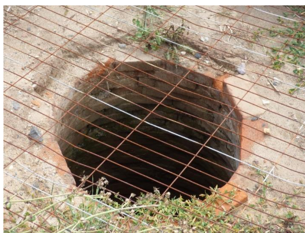
Elements of Significance include the original redbrick fabric
