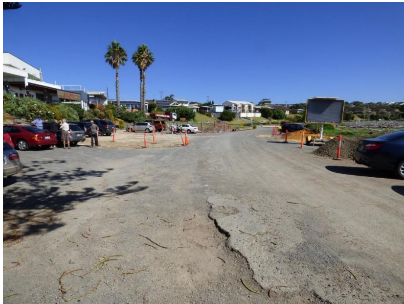
Franklin Parade prior to completion of the carpark Note location of the fenced well area towards the end of the carparking area. 17 March 2017 Source DEW
