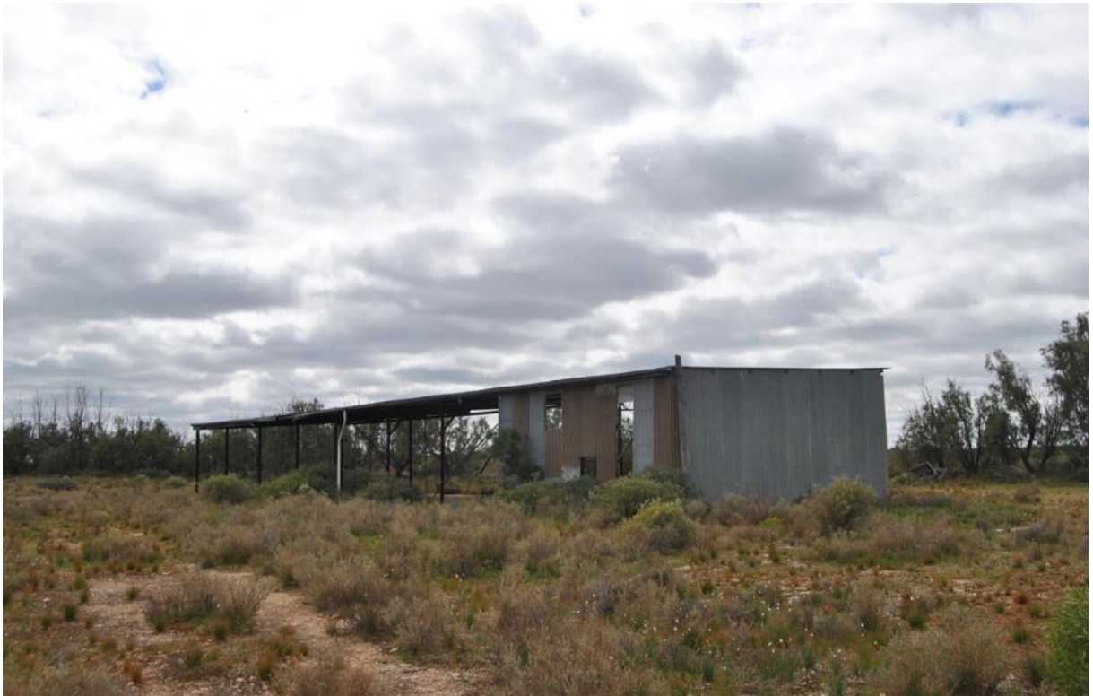
Figure 10 – Shed off Detloffs Road near quarry, looking north, 2017
