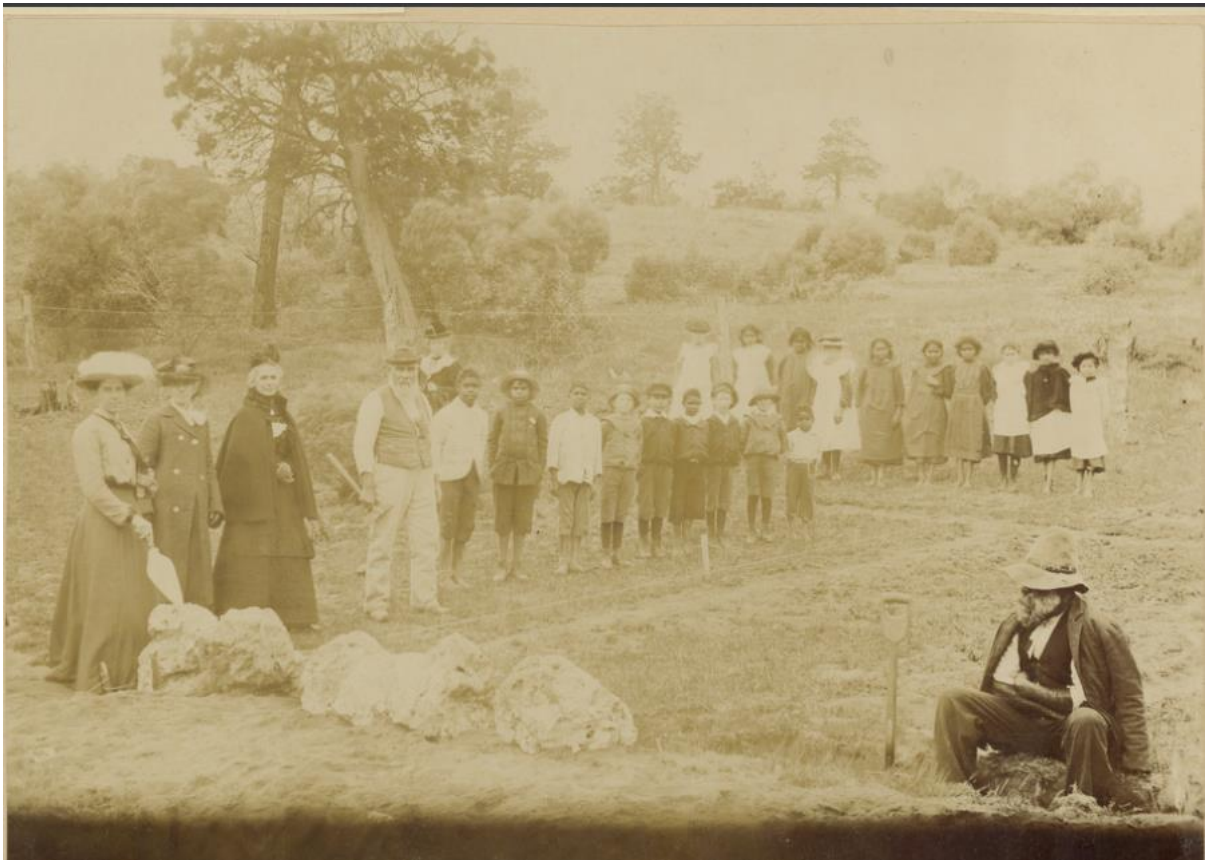
Figure 3 – Janet Matthews laying the first stone for the first building at Manunka, 1904 [Source: State Library of SA, Image No. 142/4/2/12]
