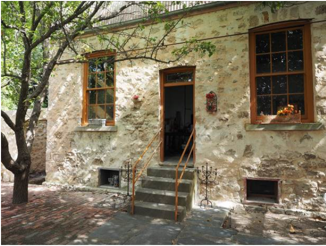
Three-storey outbuilding March 2017 Note basement level windows Source DEWNR
