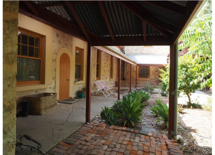
South side of Bungala House March 2017
