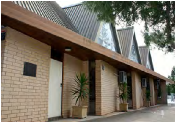
Side elevation of St Maximilian Kolbe church, October 2017. Note stepped back walls to create trapezium-shaped floor plan. Source- DEW
