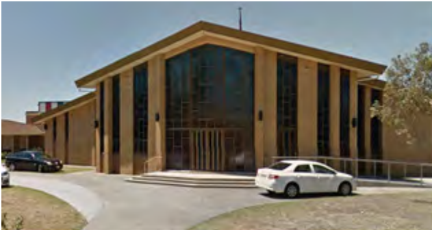
St Margaret Mary (1968), Croydon Park Source- Street view
