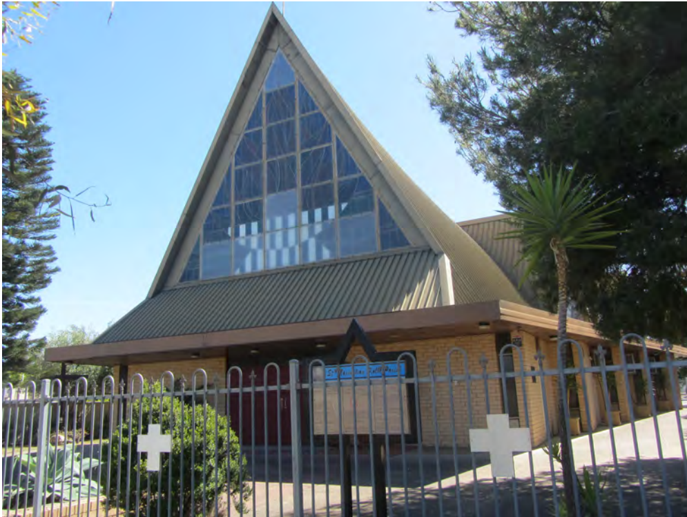
Front entrance of St Maximilian Kolbe Catholic Church, October 2017. Source- DEW
