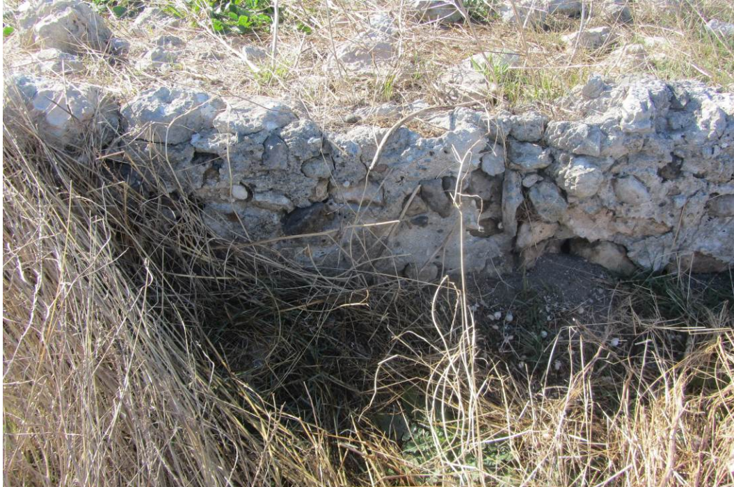
Remains of the western wall showing the fieldstone, calcrete and lime mortar
