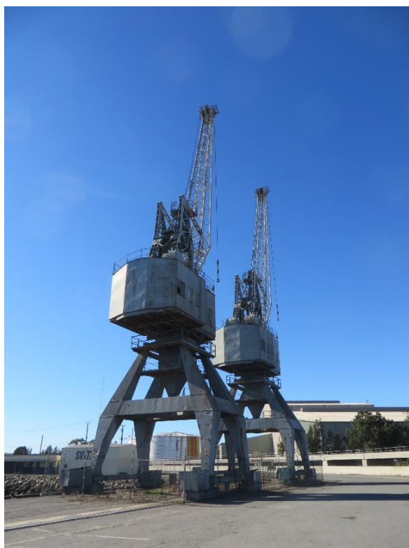
View of the surviving 2 electric cranes from the south side of No. 2 Dock (Stephen Schrapel, 2017).
