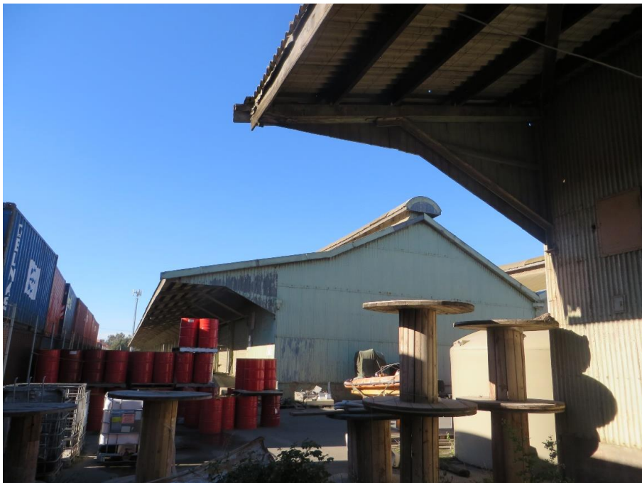
View of the Sheds 16 & 17 from the north, showing the verandah extension of the roof over a raised loading platform (Stephen Schrapel, 2017).
