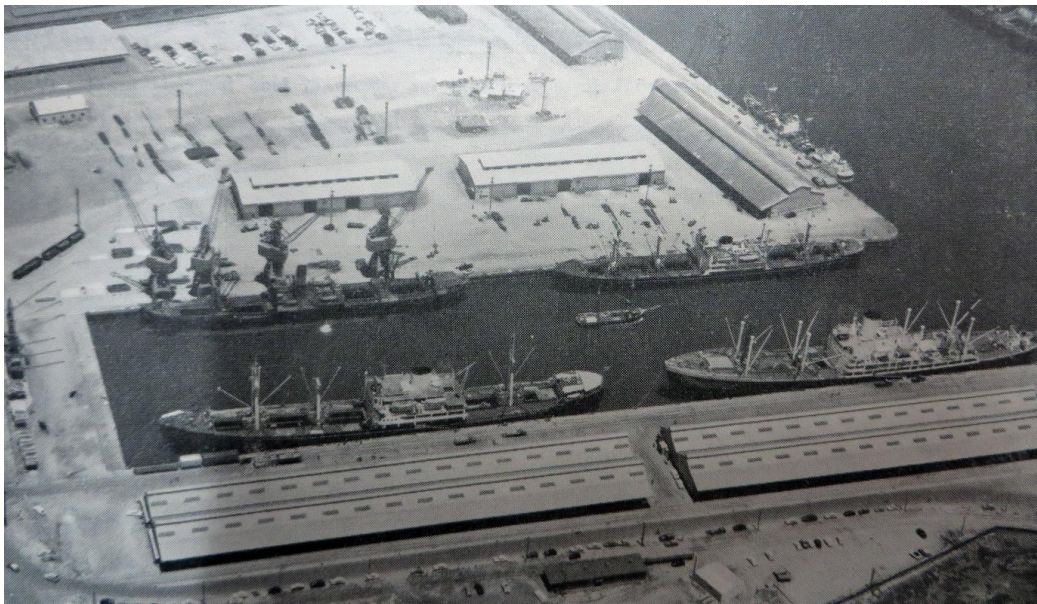
View of recently completed 13 and 14 Berths, No. 2 Dock, showing new 6-ton electric cranes, wide wharf aprons and sheds, 1959. (South Australian Harbors Board, Report of the Commissioners of the South Australian Harbors Board for the year ended 30th June 1959.)
