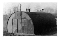
English Nissen Hut- the corrugations in the cladding run vertically and the sides flatten out at the bottom.
