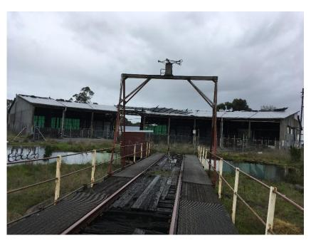
View of roundhouse and turntable showing degradation of timbers on the turntable
