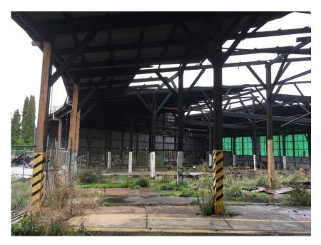
Roundhouse view to south showing intact and undamaged posts at front of structure Source: Heritage South Australia 19 July 2018
