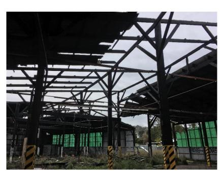
Roundhouse view to south-west showing the fire damage to the central portion of the roof frame and loss in the back wall.
