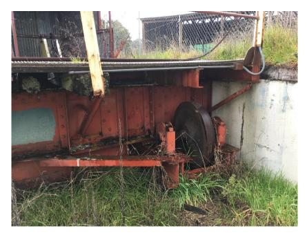
Wheel and outer rail that enabled operation without balancing the locomotives
