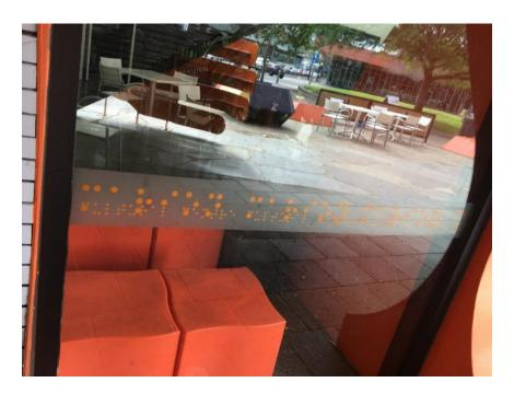
Braille panel extending along the glazing. The large dots denote 'marion', the small dots underneath denote 'cultural centre'.
