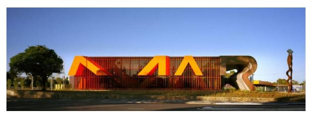
Marion Cultural Centre, north-eastern elevation facing Diagonal Road. MAR are created from a steel framework clad in steel plate, copper plate and timber batons.
