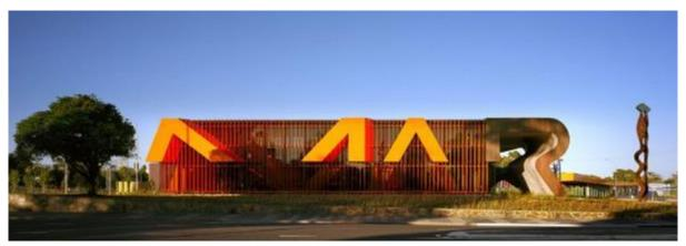
Marion Cultural Centre, north-eastern elevation facing Diagonal Road. MAR are created from a steel framework clad in steel plate, copper plate and timber batons.
