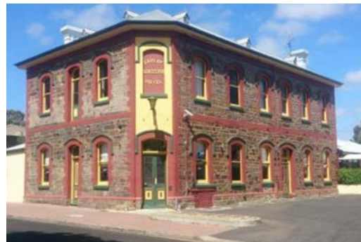
Earl of Leicester Hotel, 85 Leicester Street, Parkside, (English & Soward, architects), c.1885, (LHP)
