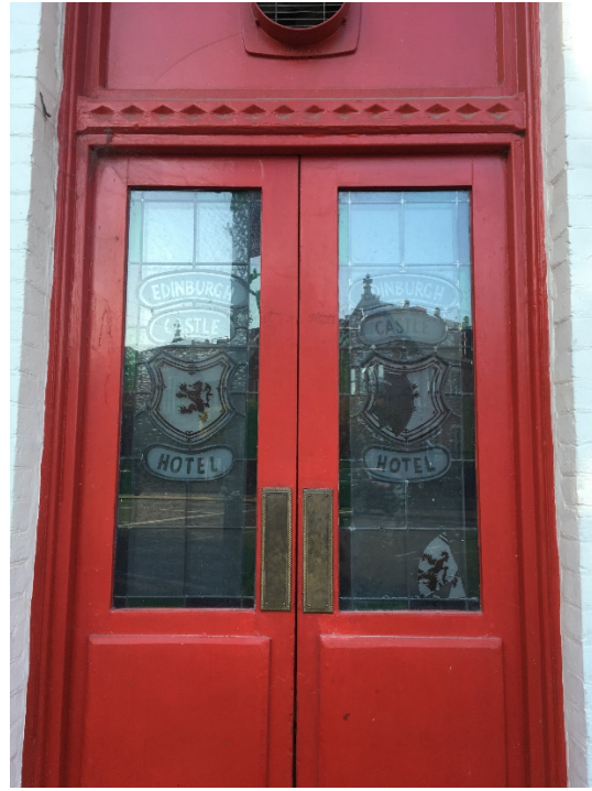
Door in chamfered corner showing the lead light
