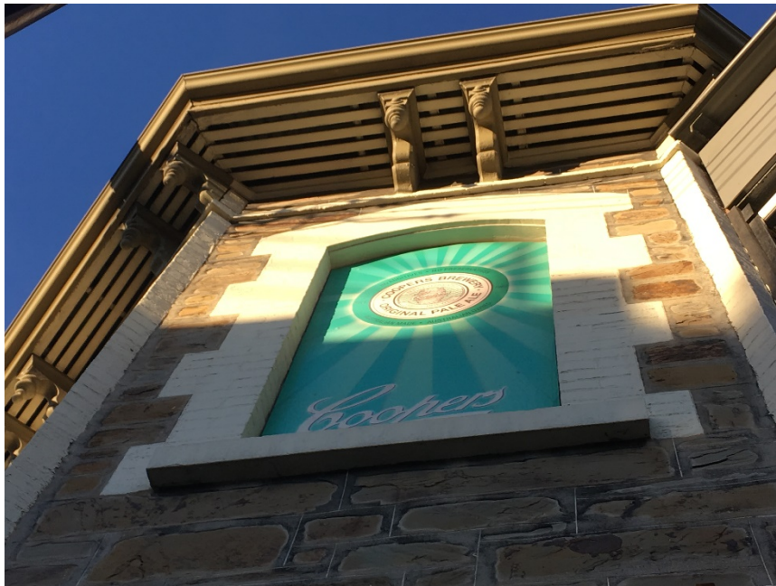
View of timber-baton, eave-soffit and decorative eave brackets
