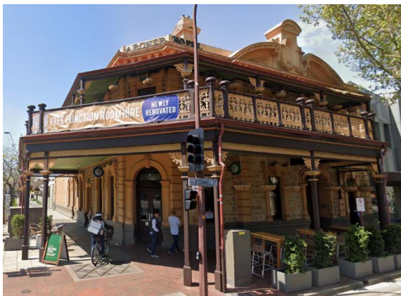
Archer Hotel (former Huntsman Hotel), O'Connell Street, North Adelaide, 1882, (SHP 13527)
