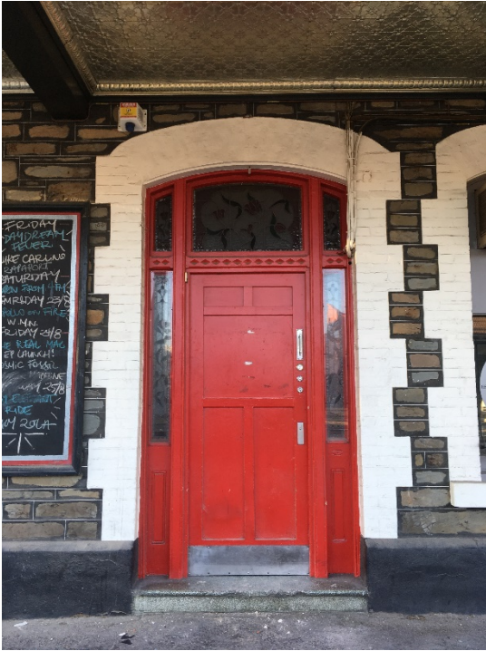
Main door to Currie Street showing the fan and slide lights
