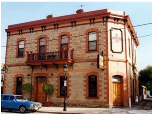
British Hotel, 58-60 Finniss Street, North Adelaide, (Rowland Rees, architect), 1882-1883, (SHP 13556)
