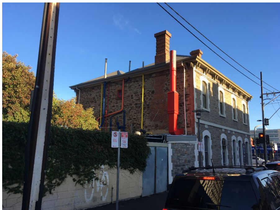
Edinburgh Castle Hotel, view of the southern and eastern elevation
