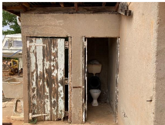
Ablutions block, toilet and shower.
