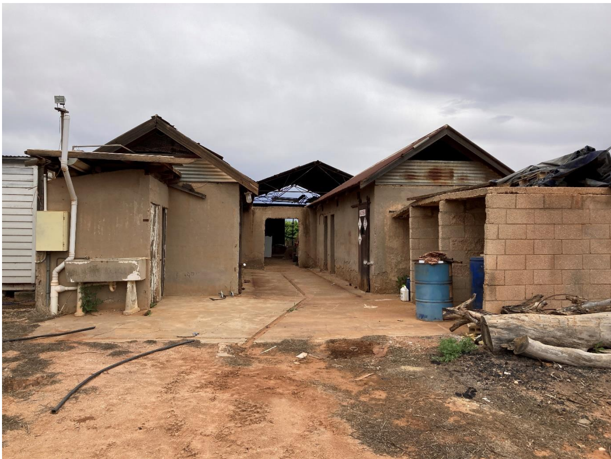
Camp 10 Cell Block, Loveday Internment Camp Complex
