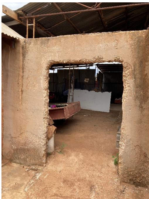
New or enlarged opening in the end wall of the cell block.
