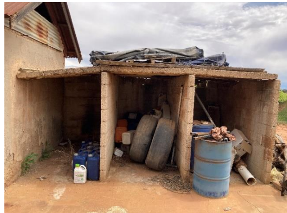
Concrete brick addition to cell block.
