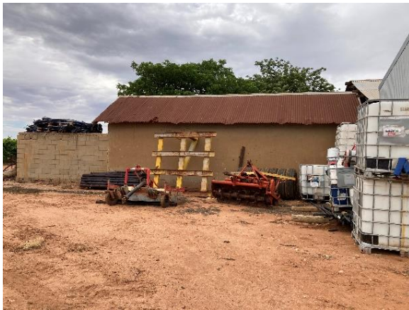
Exterior wall of the cell block.
