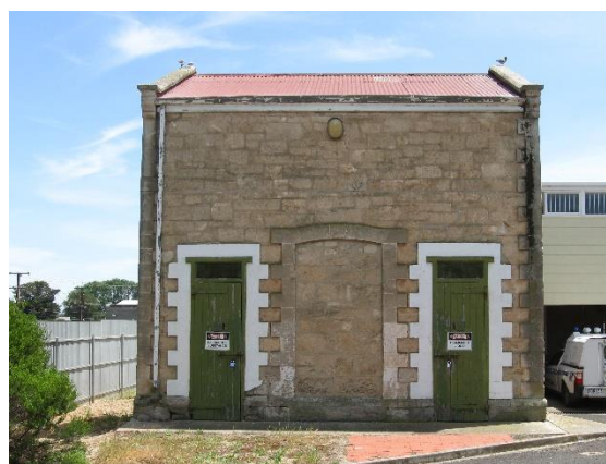
Former Lock-up Millicent Police station
