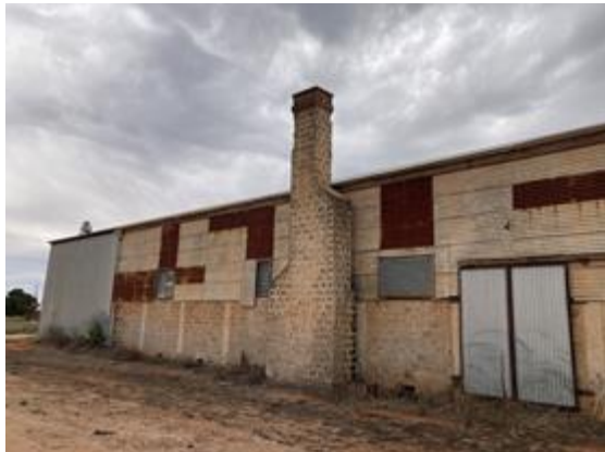
Recreation Hall, Loveday Internment Camp - General Headquarters site.
