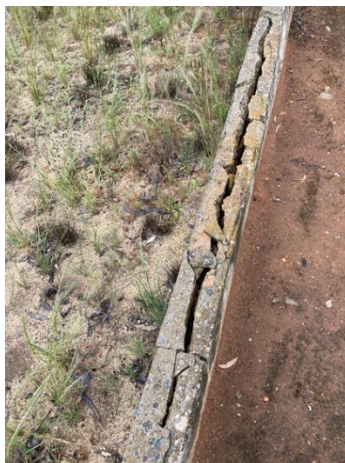
Filtration beds, showing loss of wall due to concert cancer (top).
