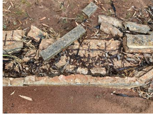
Examples of the damage being caused to the structures by spalling and jacking that will result in imminent failure.
