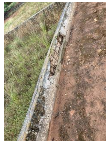
Filtration beds, showing loss of wall due to concert cancer (top).
