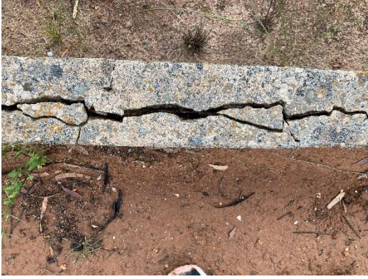
Examples of the damage being caused to the structures by spalling and jacking that will result in imminent failure.
