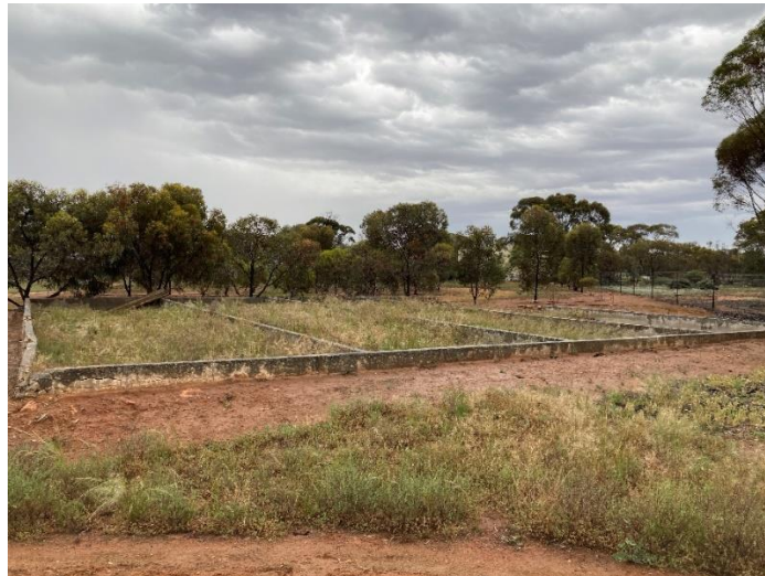
Sullage Treatment Works, Camp 14, filtration beds.
