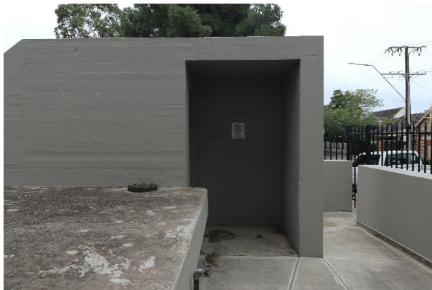
Front view showing traversed entrance DEW Files 4 February 2021
