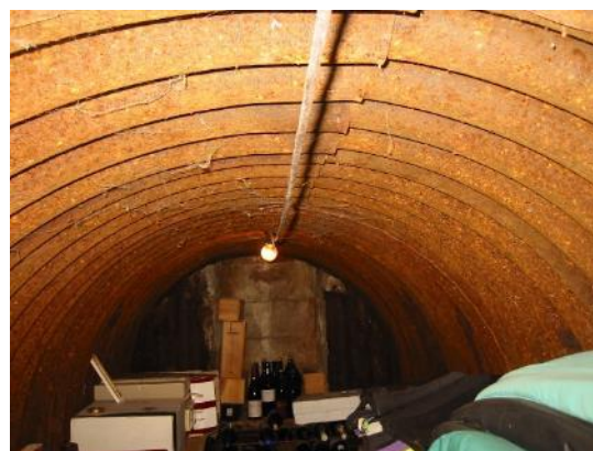
Sectional type domestic air raid shelter at 510 Greenhill Rd, Hazelwood Park
