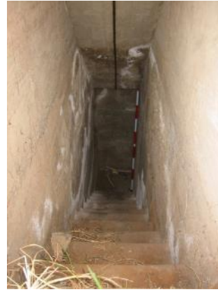
Bunker-type domestic air raid shelter at 54 Williams St Beverley
