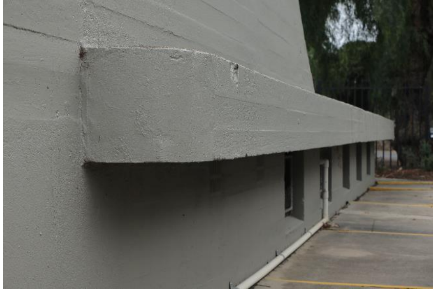
Side view showing windows DEW Files 4 February 2021
