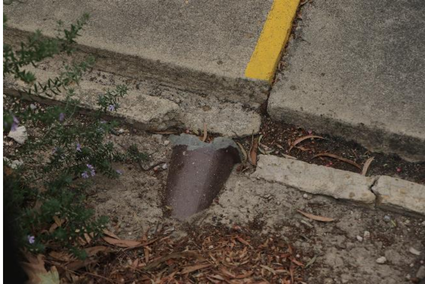
Exterior – earthenware drainage pipe DEW Files 4 February 2021
