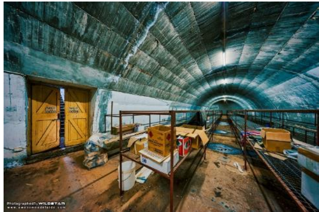
Former air raid shelter at Paternoster Road, Reid (LHP) Source: www.awesomeadelaide.com
