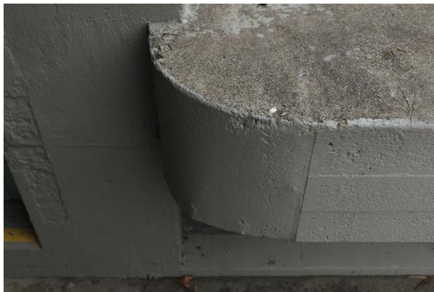
Detail of board-formed concrete DEW Files 4 February 2021
