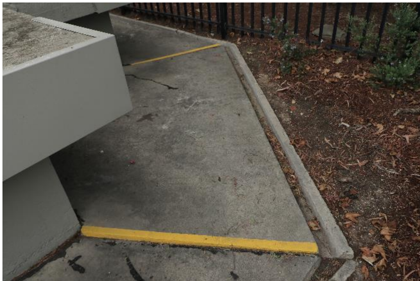
Original cement paving and integrated drain DEW Files 4 February 2021
