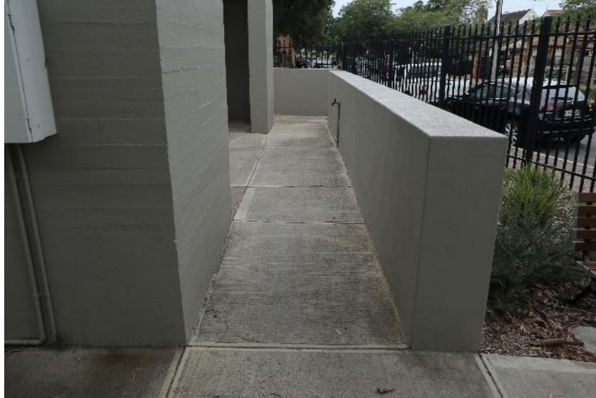
Front entrance showing baffle wall and new concrete paving DEW Files 4 February 2021
