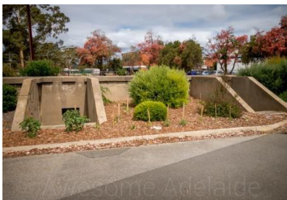
Bunker-type air raid shelter at the former British Tubemills (Australia) factory, 498 Churchill Road, Kilburn
