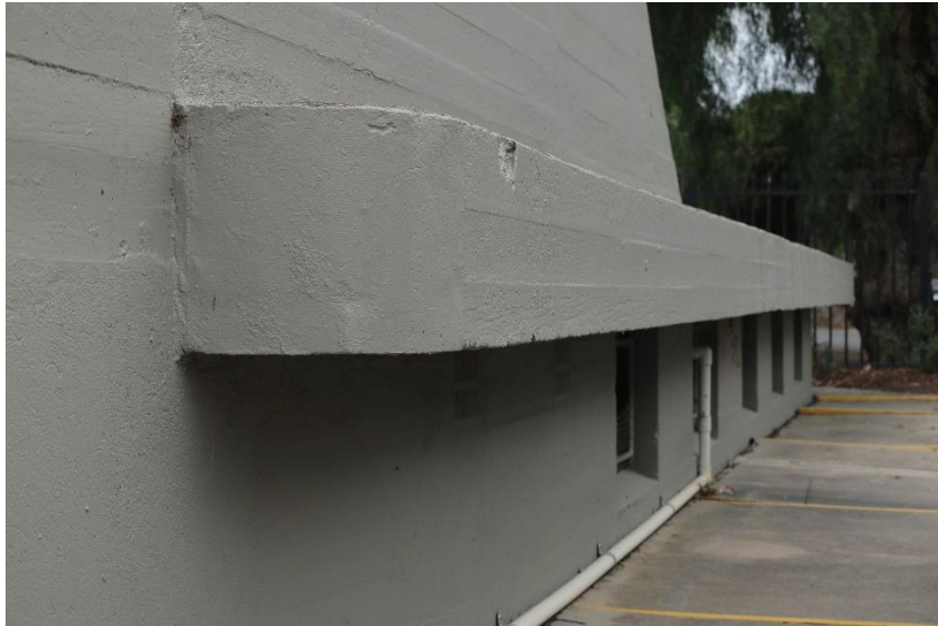
Side view showing windows
