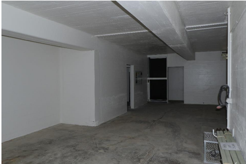
General interior view DEW Files 4 February 2021
