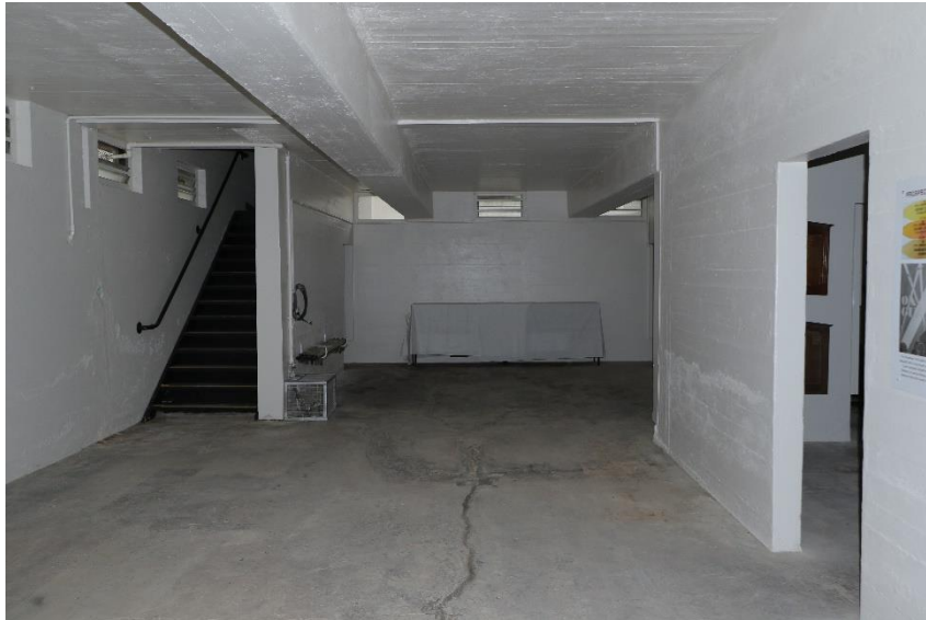
General interior view DEW Files 4 February 2021
