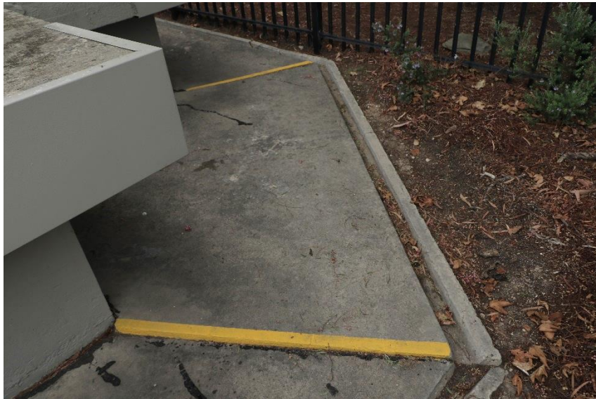
Original cement paving and integrated drain
