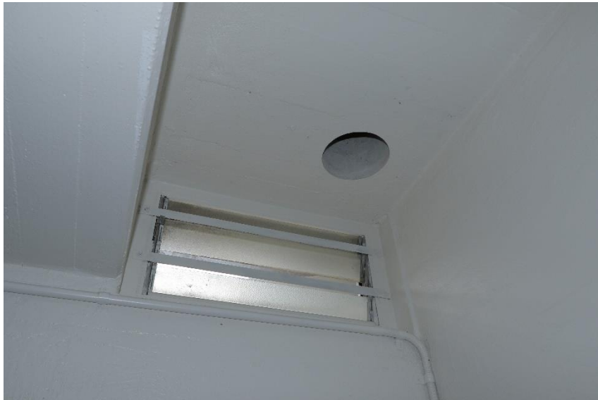
Interior view showing window and ventilator tube DEW Files 4 February 2021
