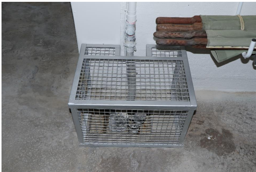
Interior view showing sump pump DEW Files 4 February 2021
