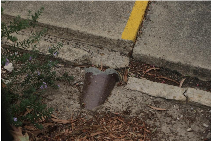
Exterior – earthenware drainage pipe
