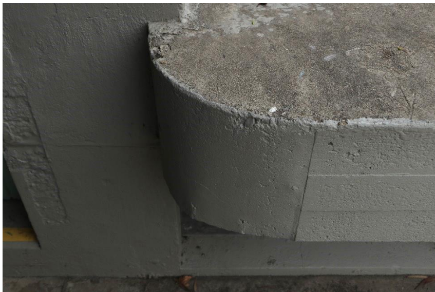
Detail of board-formed concrete
