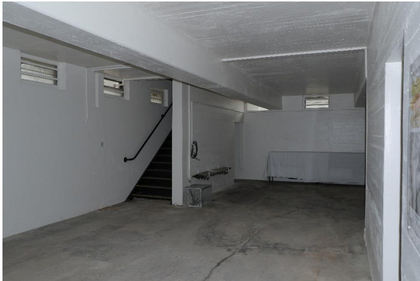
General interior view
