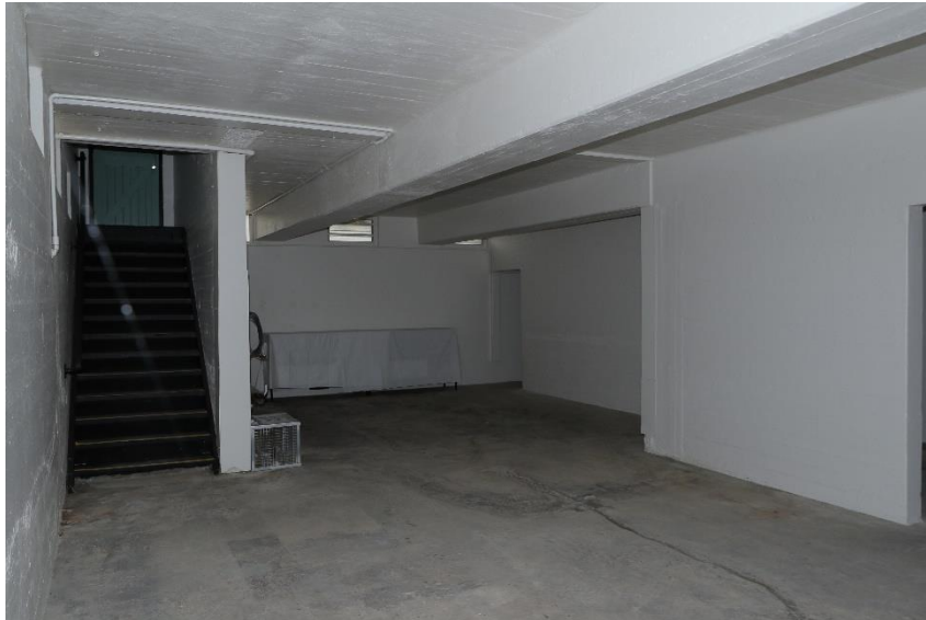
General interior view DEW Files 4 February 2021
