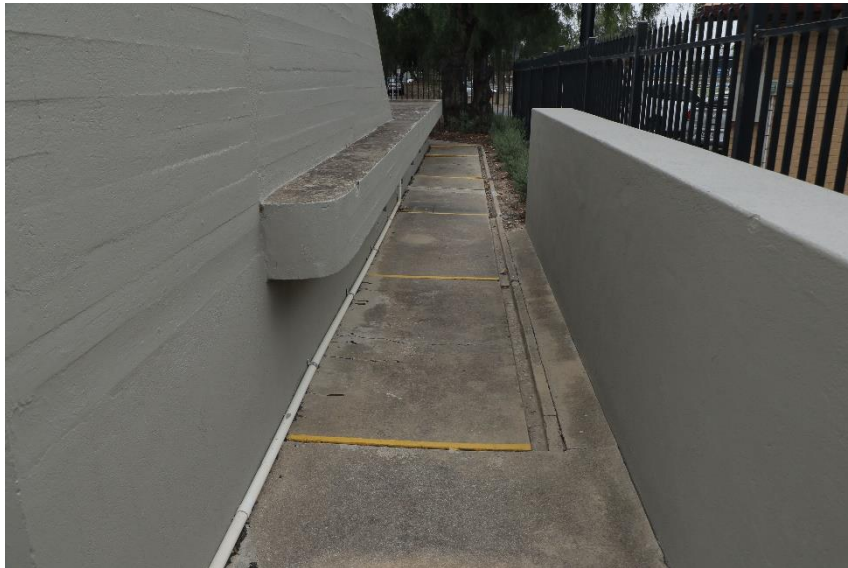
Side view showing original cement paving and integrated drain
