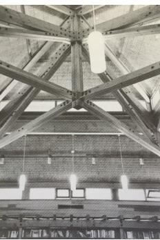
University of Adelaide Union Building (SHP 17619), showing an example of the brick grille and internal timber framing to roof and 'Solomit' compressed straw panelling to ceiling
