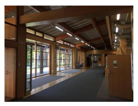
View of the front of the 1975 building, this space was once the Exhibition Hall, the wall has been slightly pushed out and replaced with glass. Note the difference in the framing between the original windows above.
