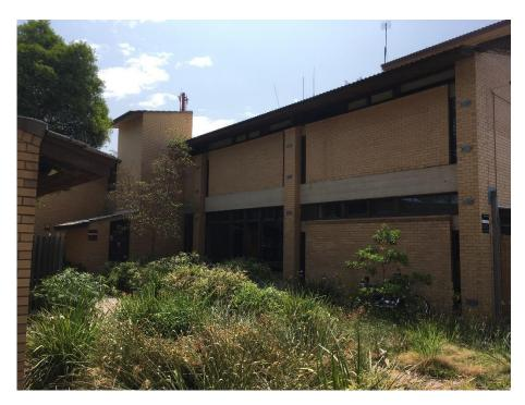
View of northern elevation showing the addition of the lift tower, off-form concrete as a decorative structural element and cream face brick.
