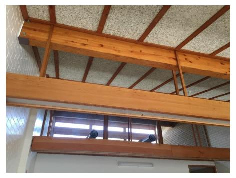
First Floor, note the 'wood wool' ceiling panels, timber beam and original bespoke light fitting that was used throughout the 1975 building.
