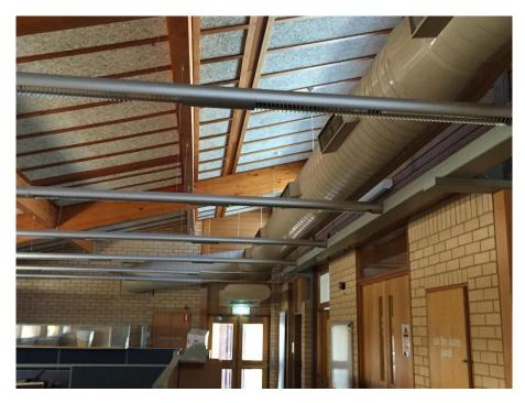
Ceiling in the 1981 addition, note the use of similar materials to the 1975 section, however, the quality of the detailing is not as high and the bespoke light fittings, which are a feature of the building are not included.
