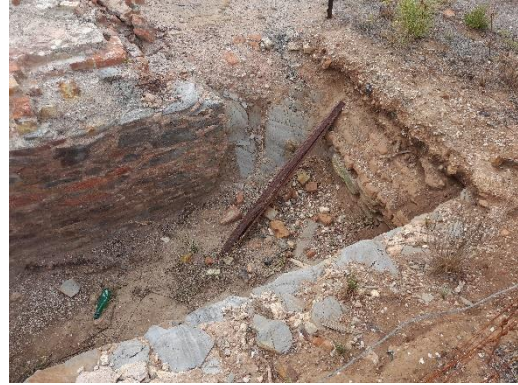
Ash pit of Smelter B
