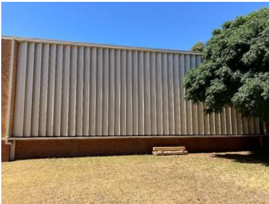
South-western side showing fixed louvres
