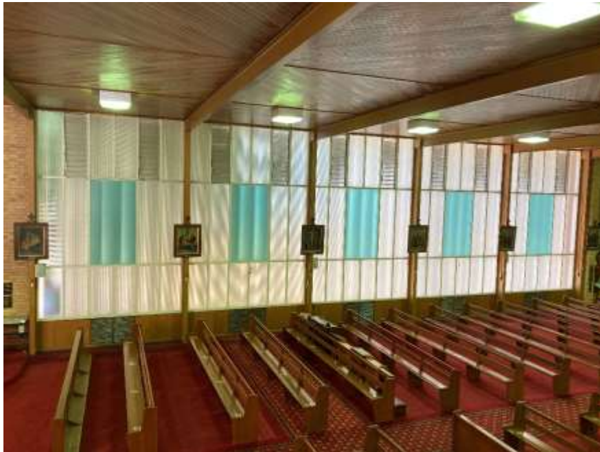
Interior view showing nave windows
