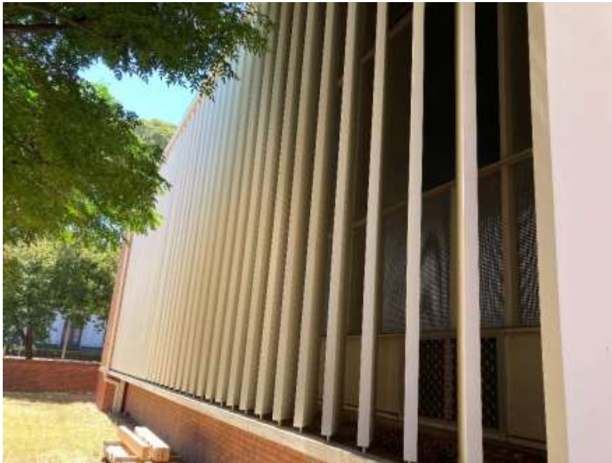
South-western side showing fixed louvres
