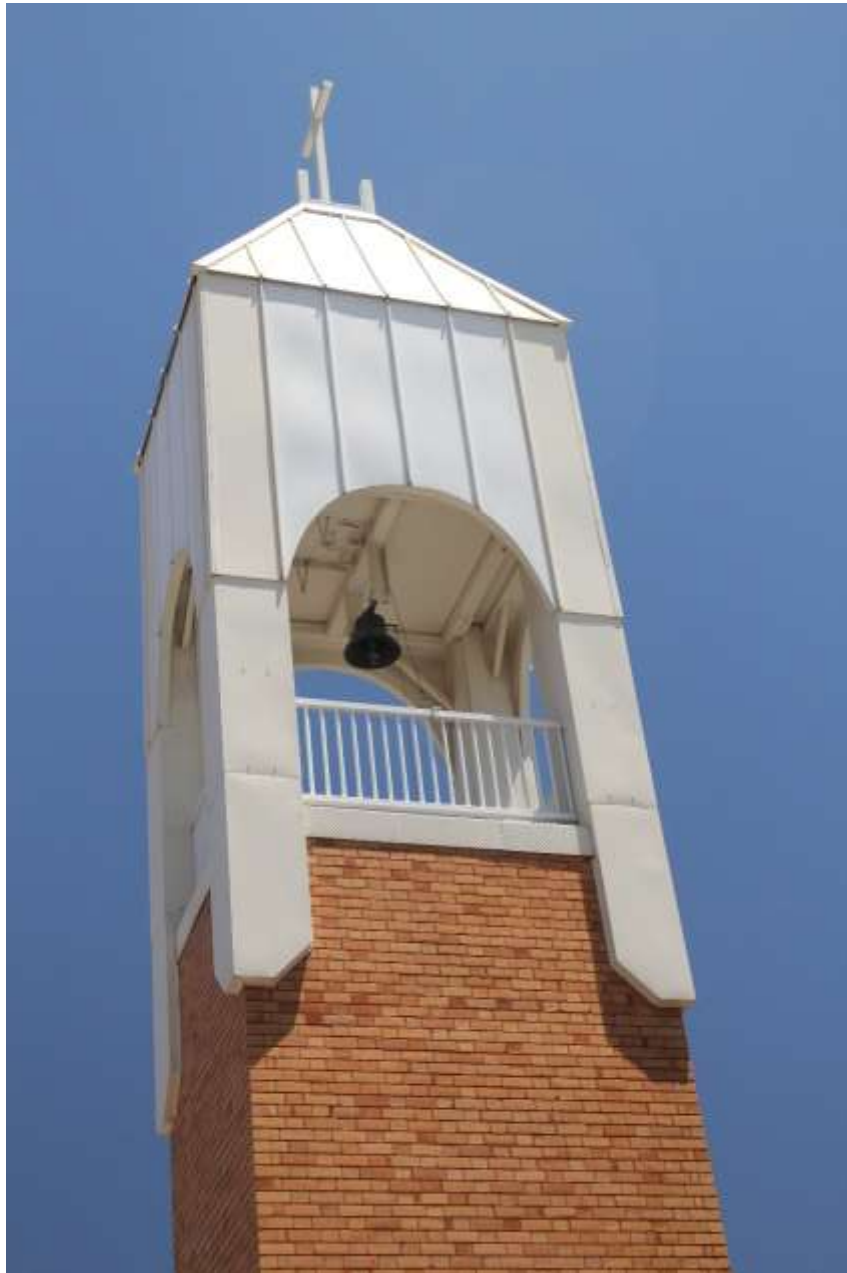
Post-1999 tower belfry
