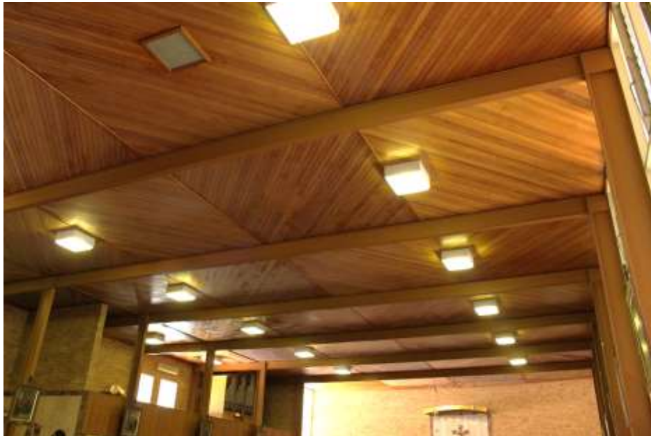
Nave ceiling showing original matchboard and replacement light fittings
