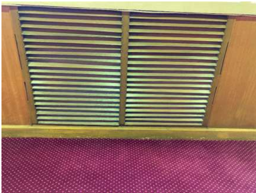
Timber louvres under nave windows
