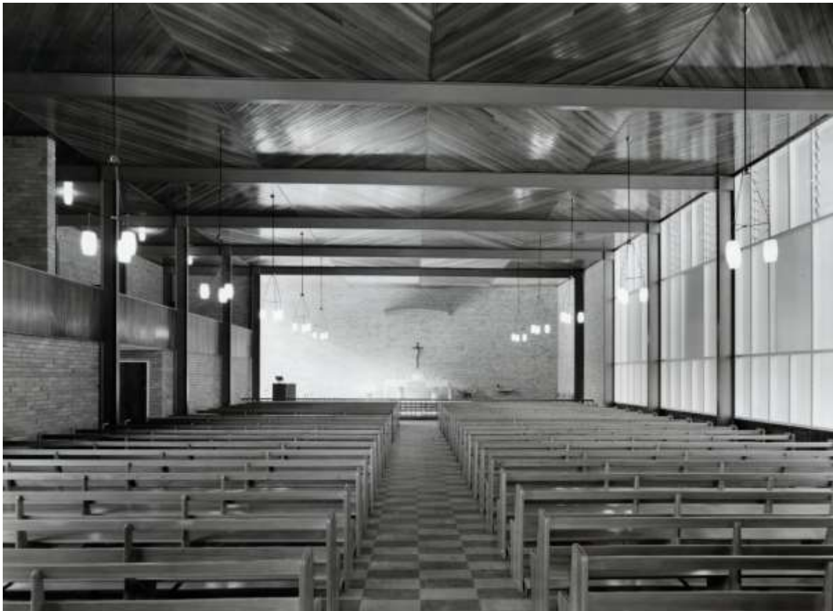
Catholic Church of the Holy Name, interior towards sanctuary, 1959
