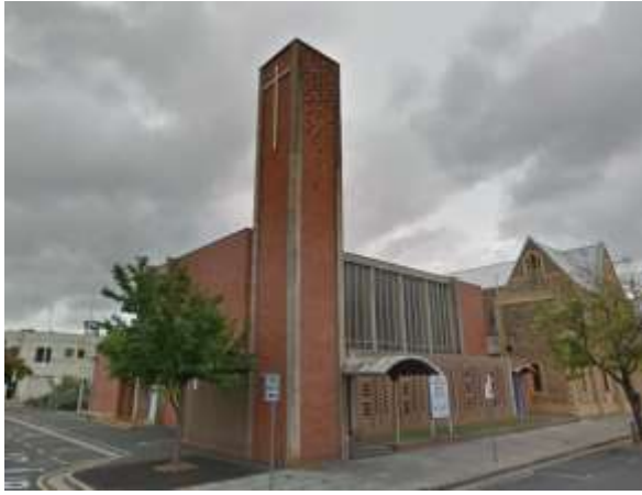
Former North Adelaide Memorial Methodist Church, North Adelaide, 1963 Source: Google Maps
