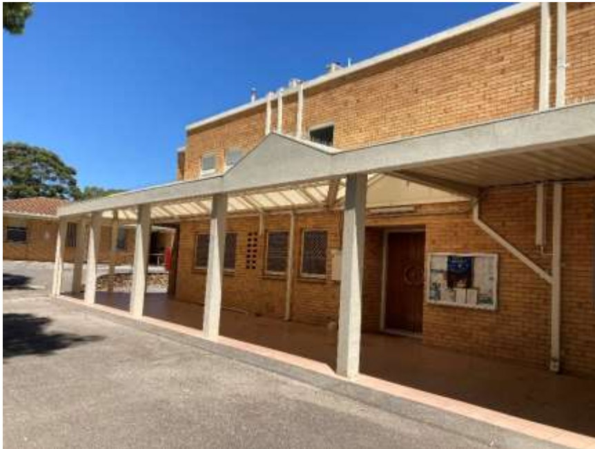
New veranda on north-eastern side
