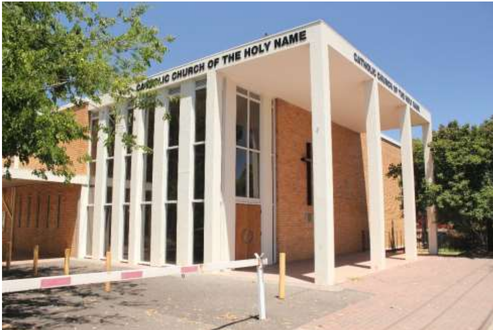
Exterior facing Payneham Road, note enclosed colonnade on left
