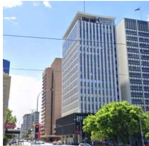
Reserve Bank of Australia now Flinders University, 1963-1967 Source: Google Maps
