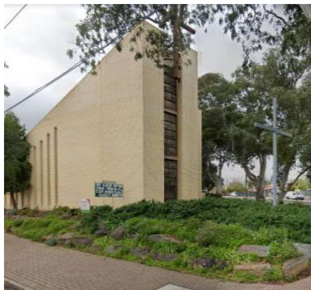
St Martin's Anglican Church, Paradise, 1971 Source: Google Street View
