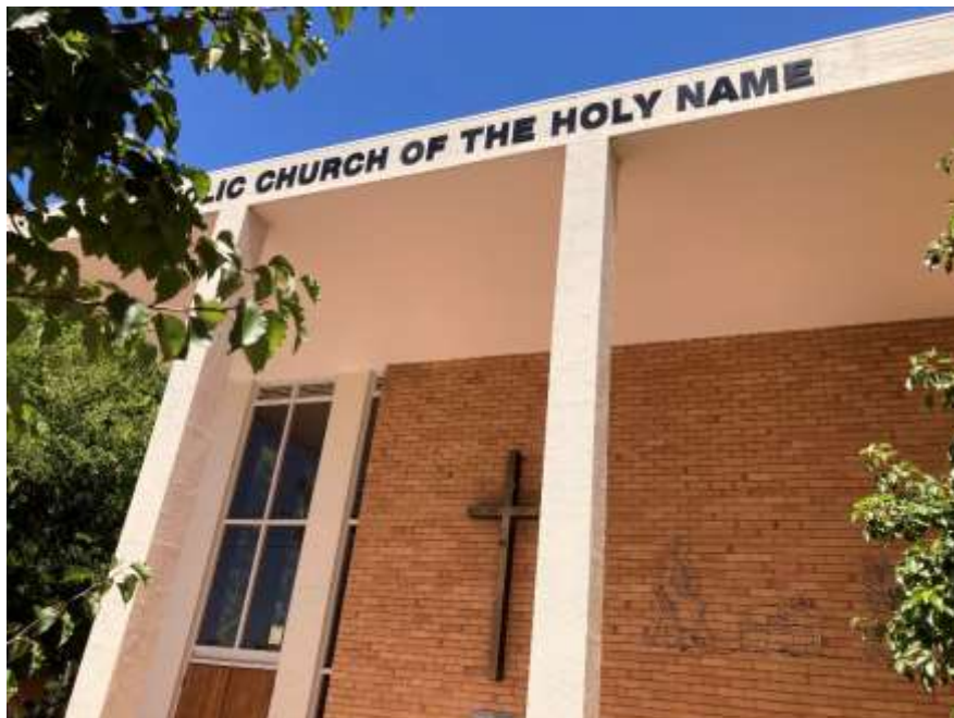
Colonnade detail facing Payneham Road
